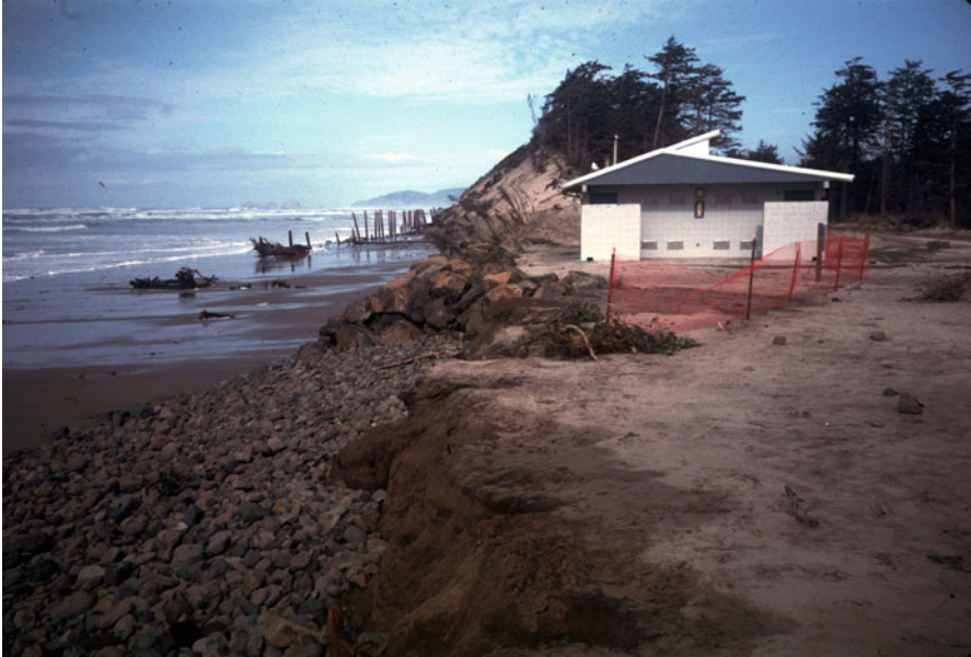
Fig. 21.17 El Niño hot spot erosion in Cape Lookout State Park on the northern Oregon coast, with the loss of its log seawall seen in the distance, leaving only the vertical supporting I-beams. Also seen is the remnant of tree-covered dunes that formerly had extended alongshore protecting the bathrooms, now being threatened by the erosion (From Komar (1986))
