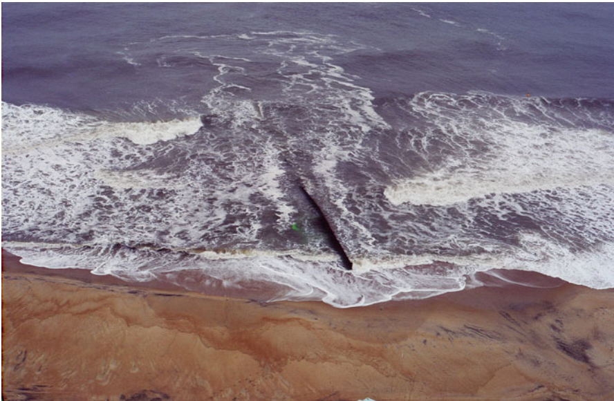
Fig. 26.8 A rip current is generated by a groin at Cape Hatteras, North Carolina (Source: S. P. Leatherman)
