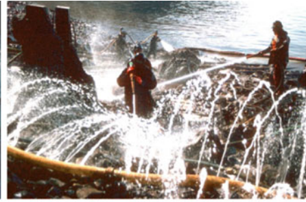
Ground view of Exxon Valdez flushing operations on heavily oiled gravel / cobble beaches.
