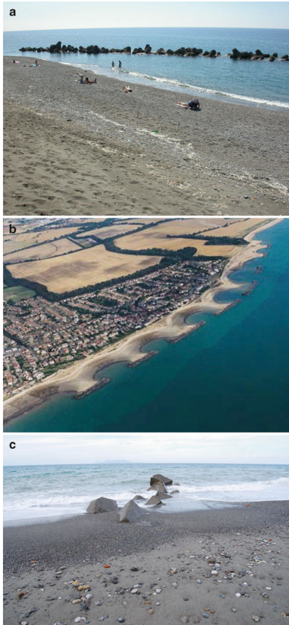
Fig. 17.3 Some examples of breakwaters: (a) in tetrapods (Italy), (b) in natural rocks (UK) and (c) in concrete blocks
