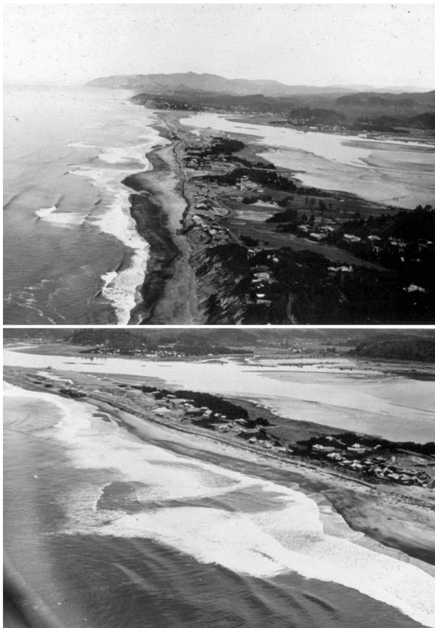
Fig. 21.14 Rip current embayments along Siletz Spit during the winter of 1972–1973, leading to the property erosion shown in Fig. 21.15 (From Komar (1997))
