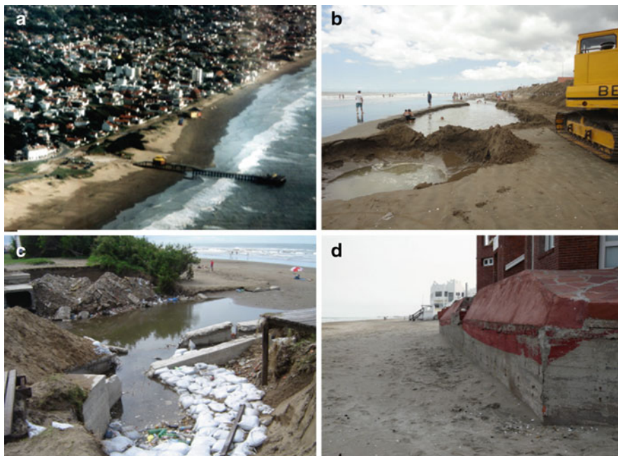
Fig. 19.14 Human direct and induced causes of erosion. (a) Effect of piers in the interruption of littoral drift, Mar del Tuyu. (b) Exploitation sand from the beach, Las Toninas, 2012. (c) Artificial fluvial discharge to the sea. (d) Seawall in the front of beach resorts, Pinamar
