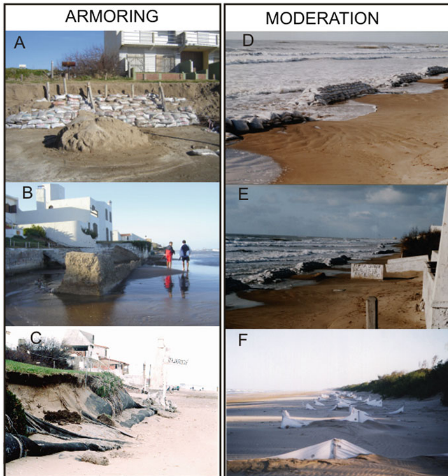
Fig. 19.17 Application of armoring and moderation classes for the dune coast of Buenos Aires. (a) Sand bags in Mar Del Tuyu for coastal protection. (b) Concrete seawalls. These rigid structure do not stop coastal retreat and collapse by undermining. (c) Geotubes. They also collapsed by wave undercutting and are very degradable with sand radiation. (d, e) Sand bags for foreshore restoration. (f) Membrane fences for backshore reconstruction
