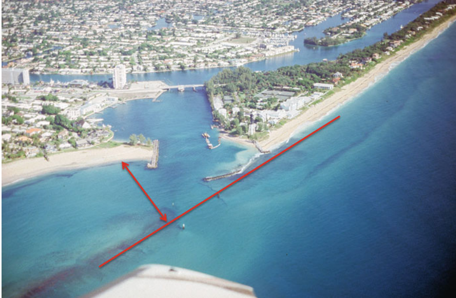
Fig. 1.2 Oblique aerial photograph of Hillsboro Inlet showing the downdrift shoreline offset. The former shoreline is marked by the shore-parallel line and the relative amount of shoreline recession (erosion) is shown by the shore-perpendicular line with double ended arrows , marking a distance of about 230 m. When the inlet was first stabilized by jetties, it became a littoral drift blocker and the downdrift beach became starved of bypassing sand. Today, the littoral drift is stabilized by a weir jetty and a floating dredge that bypasses sand from an updrift sand trap to the south side of the inlet (Photograph by C.W. Finkl)
