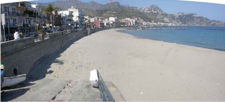
Fig. 17.4 Example of soft engineering protection: Nourished beach (Giardini Naxos – Sicily – Italy)
