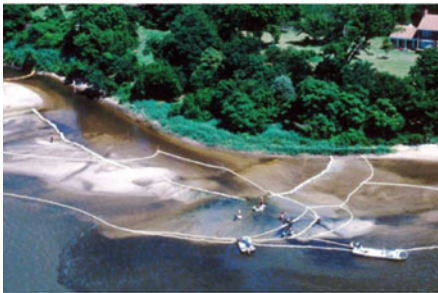
Overview of sand flushing activities with sorbent booms, Swanson Creek spill, Maryland, USA.
