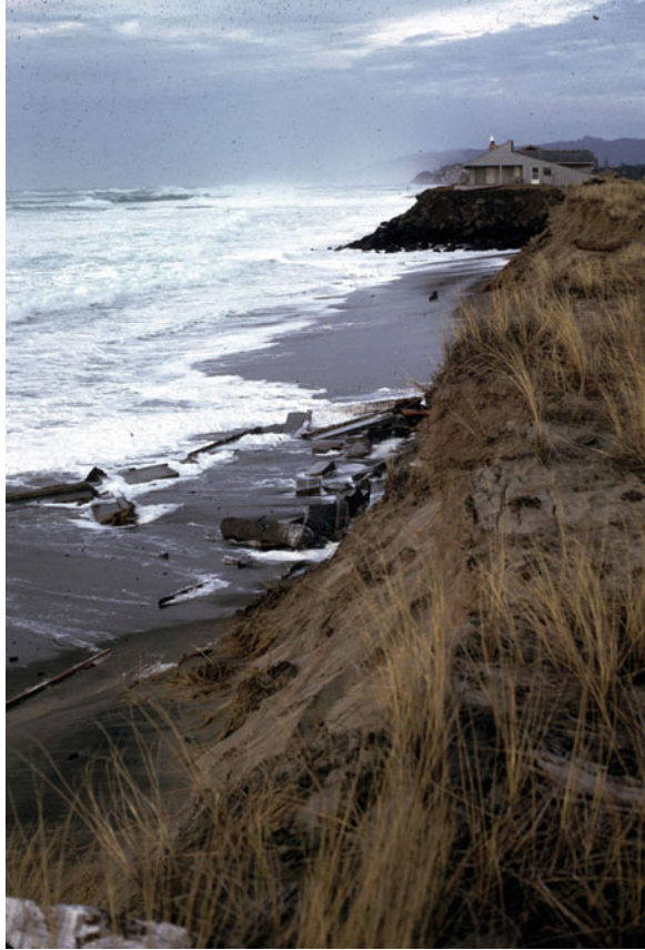
Fig. 21.15 A house under construction lost to the 1972–1973 erosion of Siletz Spit, and a house protected by a riprap revetment (From Komar (1997))
