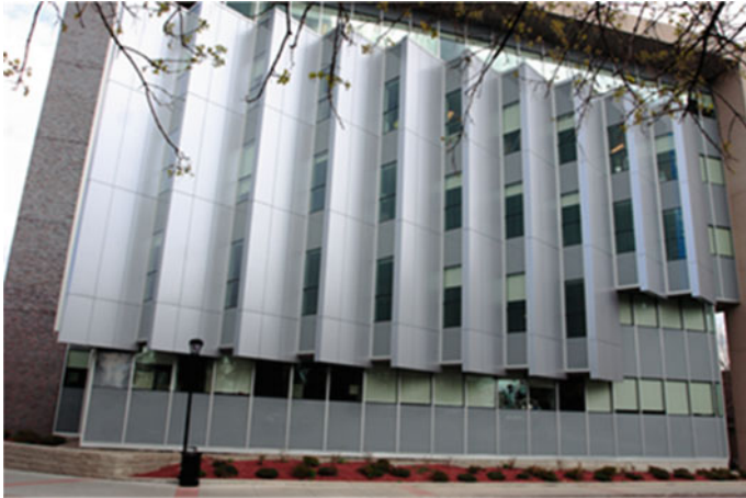
Fig. 6.20 West-facing façade of monitored building
