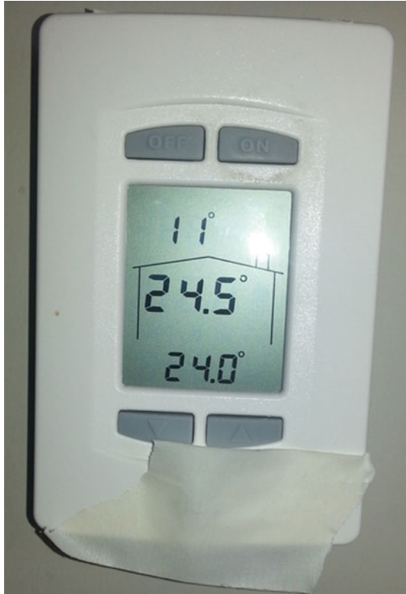
Fig. 6.16 Example of intentional sensor obstruction, where the occupant covered the PIR sensor with masking tape
