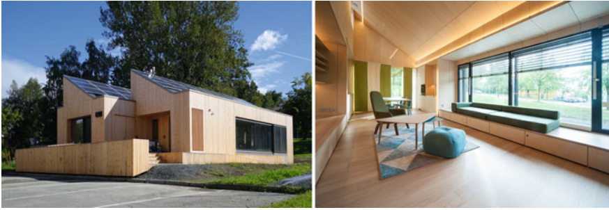
Fig. 7.9 Exterior view ( left , photo by Katrine Peck Sze Lim, NTNU) and main living room ( right , photo by Anne Jørgensen Bruland, NTNU) of the ZEB Living Lab
