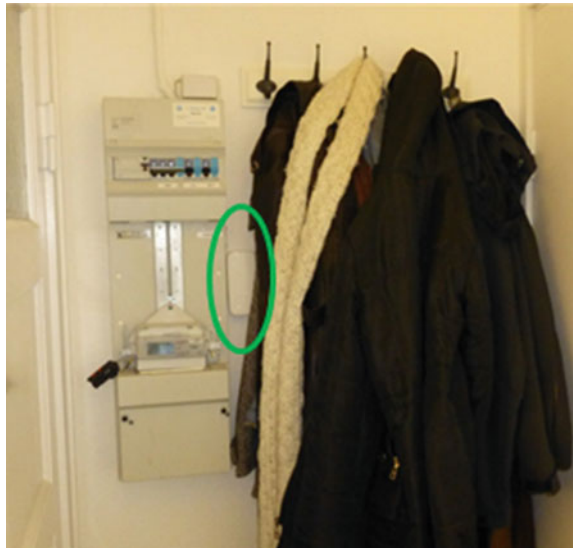
Fig. 6.17 A packaged temperature, relative humidity and CO 2 concentration sensor that was subsequently covered by coats (Andersen 2013)
