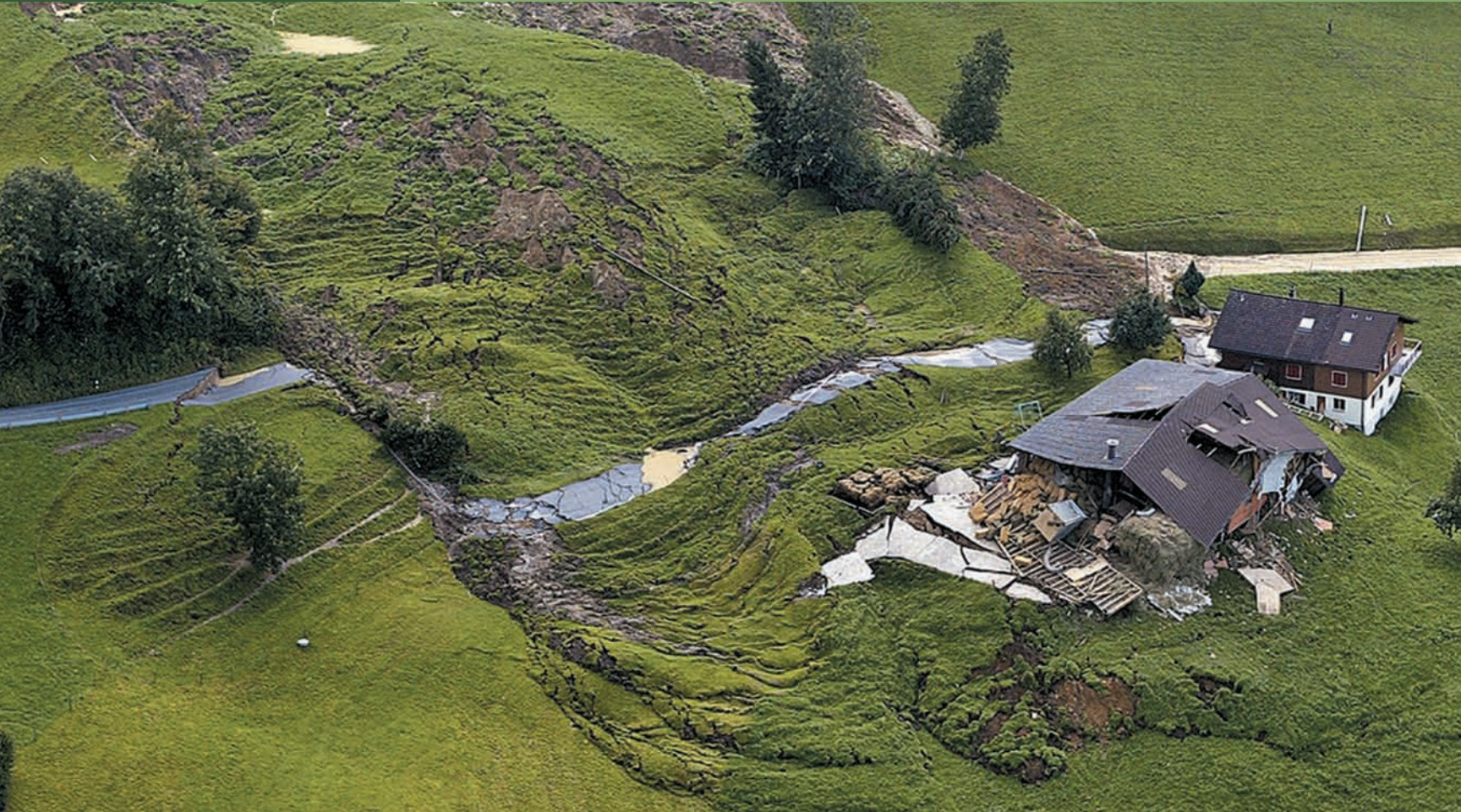
A farm house and stable are damaged by a landslide outside the town of Entlebuch, central Switzerland, Tuesday, Aug. 23, 2005. Note the displaced segment of the road. This landslide is an example of a slump-earthflow described in this chapter. Photo © AP/Wide World Photos
