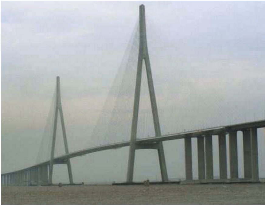
Figure 1. The Sutong Bridge is currently (in 2011) the world's longest span cable-stay bridge. It spans the Yangtze River between Nantong and Changshu in the People's Republic of China. It has a main span of 1,088 metres, and two side spans are 300 metres each, and there are also four small cable spans. Photo credit: Wikipedia.
