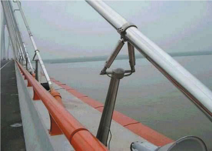
Figure 10. Semi-active vibration reduction on the Dongting Lake Bridge, which is a cable-stayed bridge crossing the Dongting Lake where it meets the Yangtze River in China. The cables were observed to have rain-wind-induced vibration, especially under adverse weather conditions and so a magnetorheological (MR) damping system was introduced to reduce cable vibration. Here you can see how the pair of MR dampers, at an inclined angle are attached to the cable. Photo credit: Wikipedia.
