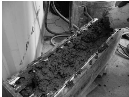
Figure 6. Casting procedure for configurations 1, 2 and 4 – concrete poured through the connectors.
