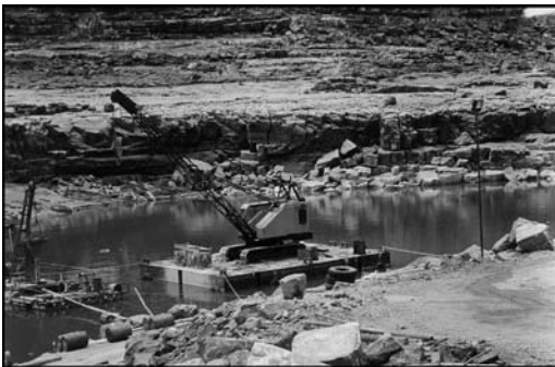
Figure 5. Placing of Gabion Shuttering in progress.
