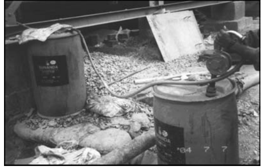
Figure 7. Dosing of Sunplast AWA to batching plant.
