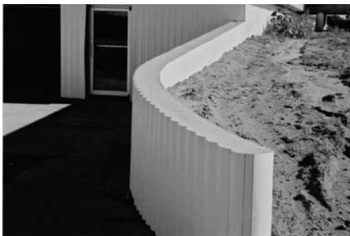
Figure 1. Retaining wall encased with PVC stay-in-place formwork.
