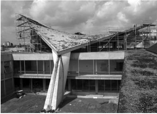
Figure 1. Steel reinforced concrete hyper-shell of FH Schweinfurt.
