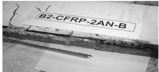
Figure 8. Complete CFRP cutting-off at the middle span of beam.
