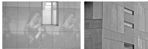
Figure 1. Ventiladed façades (DIBt 2004, Engberts 2006).
