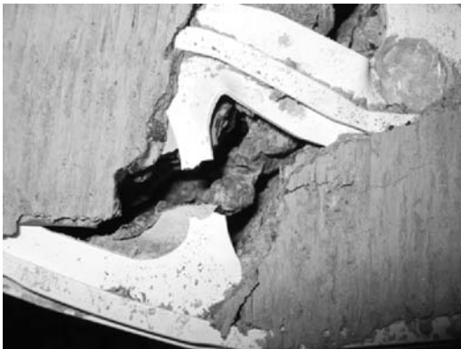
Figure 17. Weakest-point of PVC-encased specimen after 7 mm deflection.
