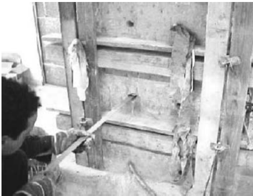
Figure 3. Column confinement with AFRP rods.
