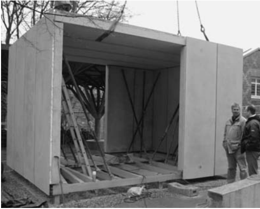
Figure 10. Assembly of modular prototype sandwich building.
