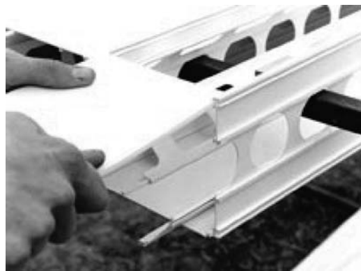
Figure 2. PVC stay-in-place formwork cell assembly.
