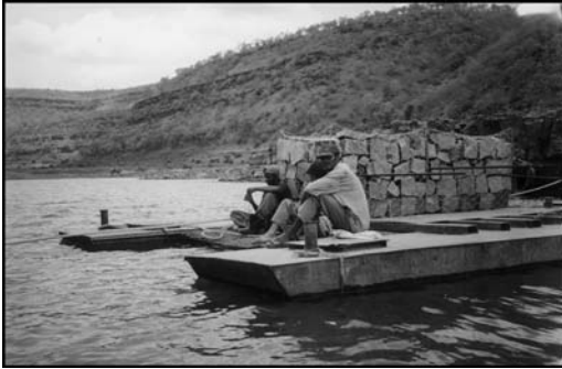
Figure 4. Gabion Shuttering.
