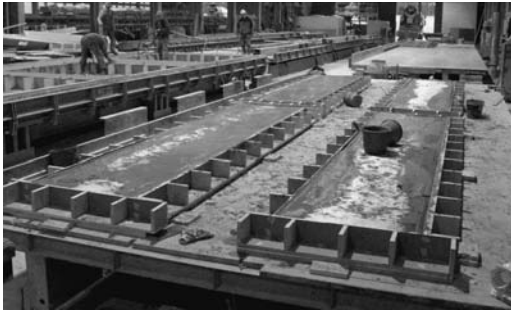
Figure 14. Casting of modular roof panels in precast plant.
