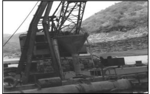
Figure 8. Gabion Shuttering.
