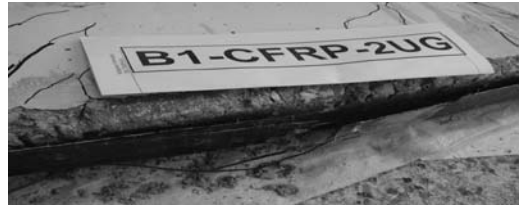
Figure 7. CFRP cutting-off at the middle span of beam.
