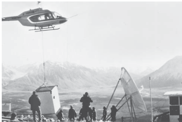
Figure 14.7 Transportable message station. (Courtesy of Telesat Canada, 1983.)
