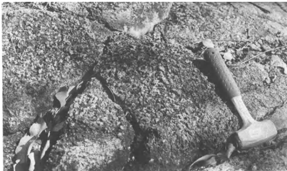
Fig. 3.19. Pitting at Mt Bunday, near Darwin, N.T.
