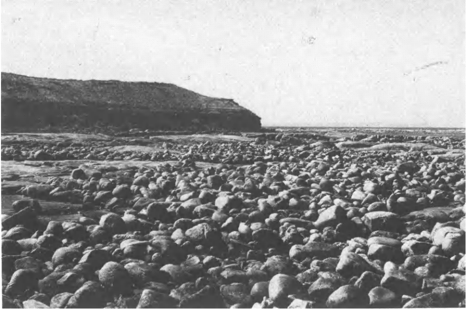
Fig. 1.7. On the west coast of Eyre Peninsula the unconformity between Precambrian rocks (commonly granite, but also including gneisses) and Pleistocene dune calcarenite frequently occurs within the present tidal and spray range. As a result the weaker limestone has in places been stripped away, as has the grus developed at the granite surface. The exposed weathering front, together with the boulders (corestones) released by the evacuation of the grus, now forms shore platforms strewn with boulders and of a width unusual for granitic environments. This example occurs just south of Streaky Bay.
