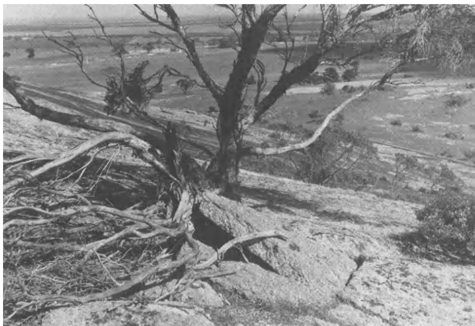
Fig. 11.27. During their growth the roots of this tree, on the upper slopes of Mt Wudinna, have displaced slabs, some of which weigh roughly half a tonne.
