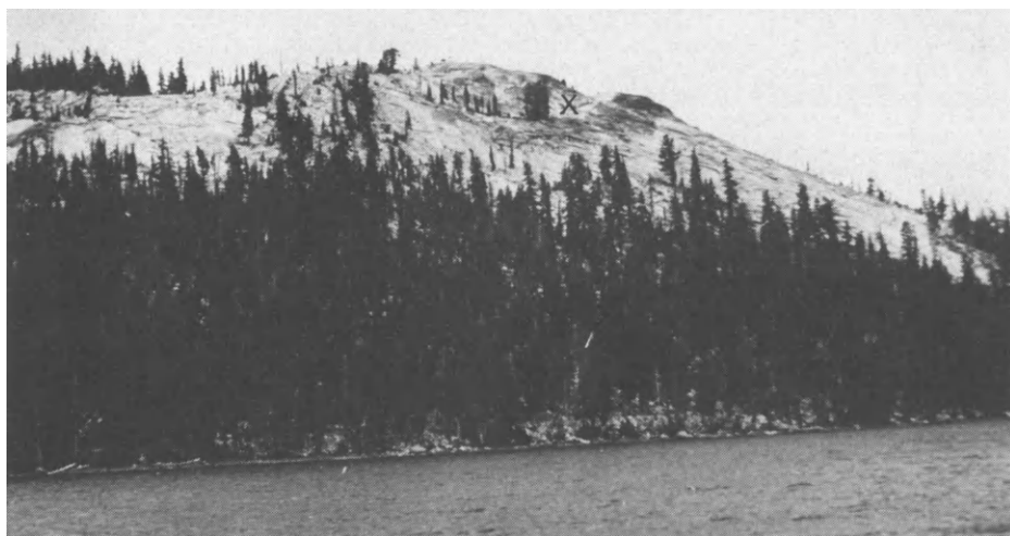
Fig. 2.30. This low dome near Tenaya Lake, Yosemite Valley, California, is apparently underlain by arcuate fractures (X) of synformal geometry.
