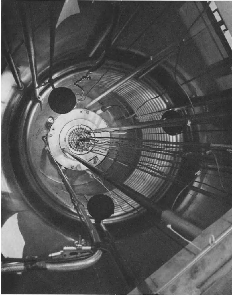
Fig. 9. Photograph of TRIGA Mark I reactor, looking down at core through the water pool
