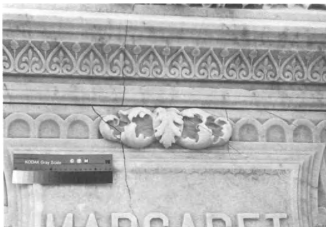
Figure 6. Deeply Carved Area of Sculpture After Biocidal Cleaning Treatments. Refer to Figure 5 for comparison.
