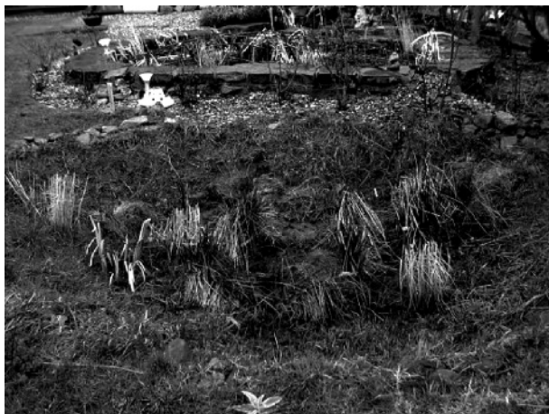
Figure 1.5 Experimental ponds located near Bradford, UK, for treating roof runoff
