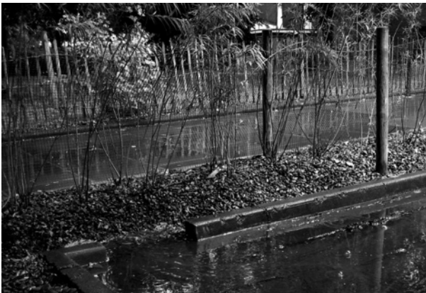
Figure 4.21 Example of an experimental belowground detention tank (below the foot path) receiving runoff partially treated with willows
