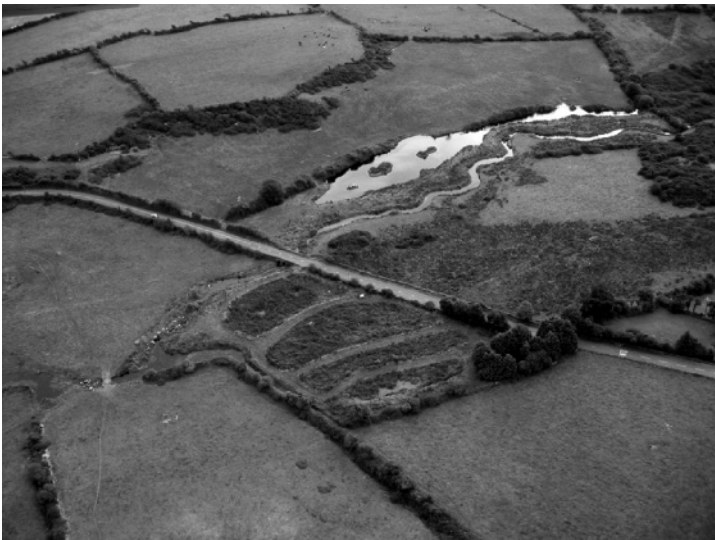
Figure 2.4 Integrated constructed wetland system in Dunhill, near Waterford, Ireland
