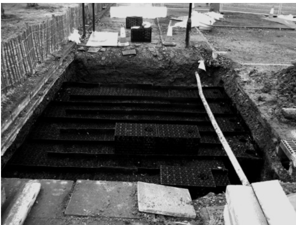
Figure 4.18 Practical application of plastic crate-based detention system
