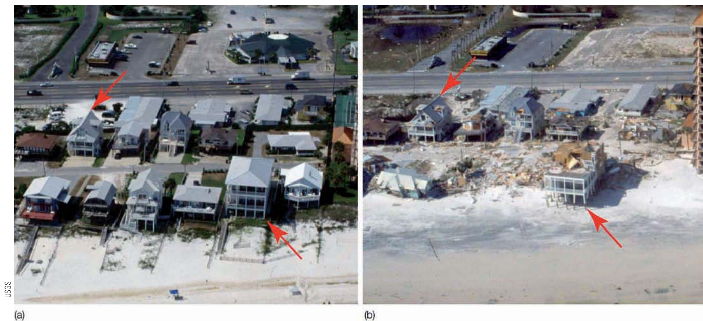
● FIGURE 15.22 Beach homes along the Gulf Coast at Orange Beach, Alabama (a) before, and (b) after Hurricane Ivan made landfall during September, 2004. (Red arrows are for reference.)
