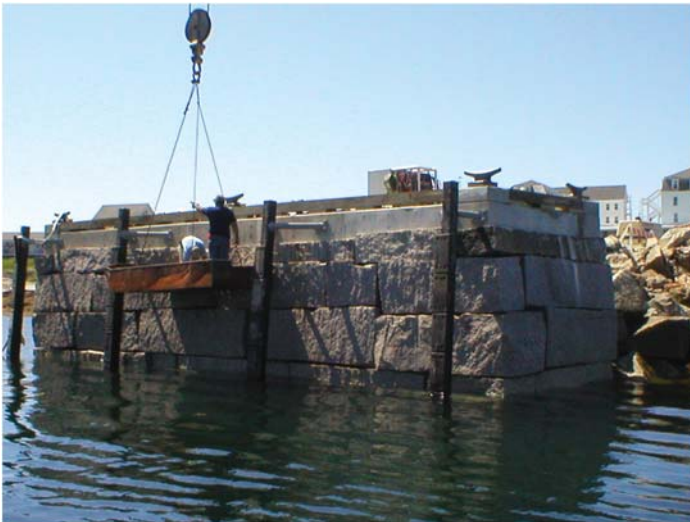
Fig. B-24. Typical masonry structure under construction
