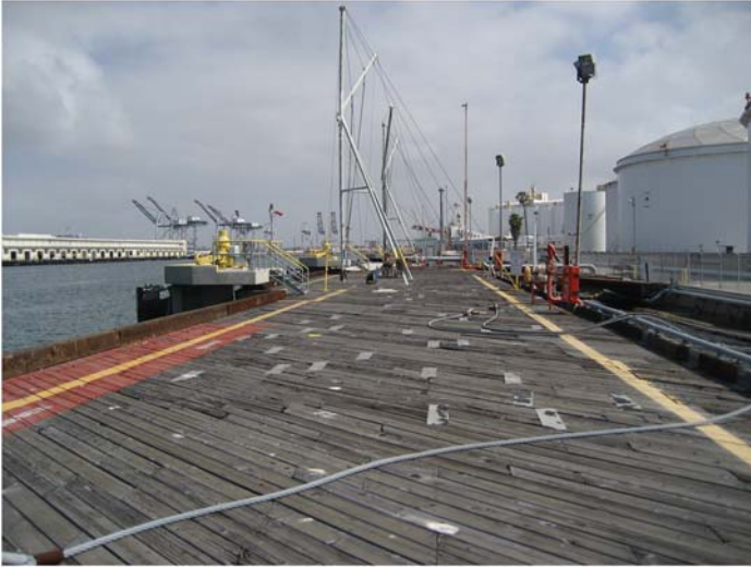
Fig. A-6. The deck of a typical timber wharf; note the numerous steel patches placed over worn, damaged, or deteriorated deck locations
