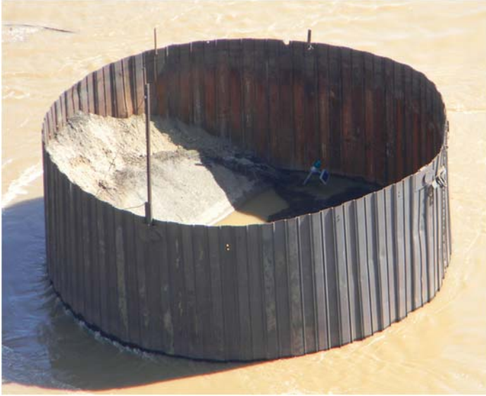
Fig. A-26. Collapse of the concrete cap due to settlement of infill material Source: Courtesy of Marine Solutions, Inc., reproduced with permission.
