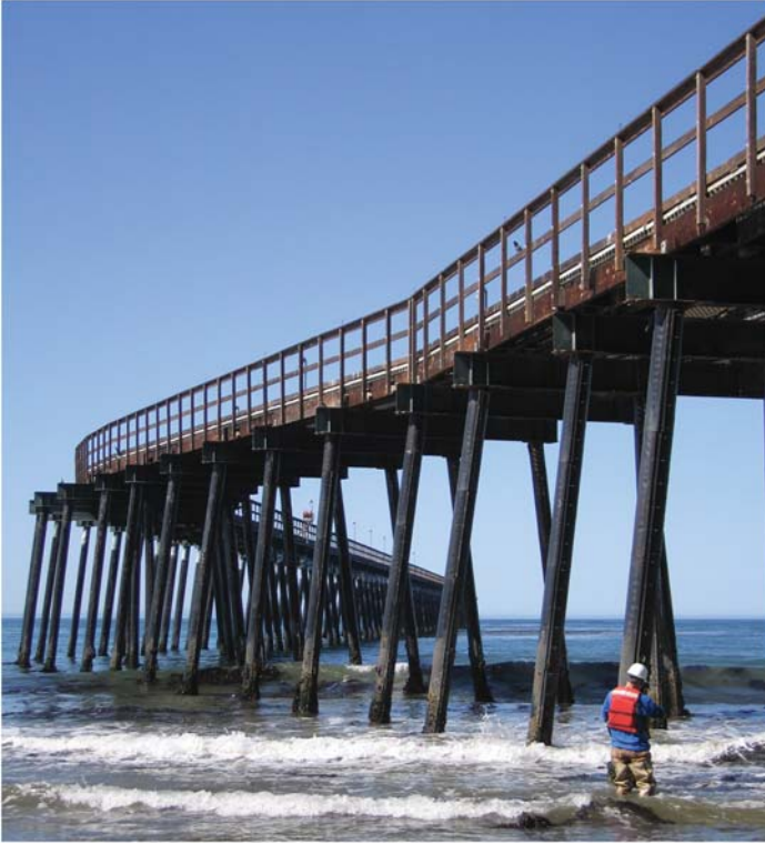
Fig. A-11. Steel ocean pier; note height of deck that cannot be adequately inspected from water or shore
