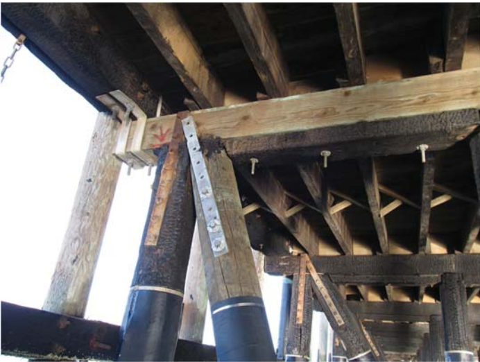
Fig. A-4. A view of the underside of a typical timber wharf. Note the stringers spanning between pile bents. Bridging is provided at midspan of the stringers to stabilize the members during installation. Source: Courtesy of Simpson Gumpertz & Heger, Inc., reproduced with permission.
