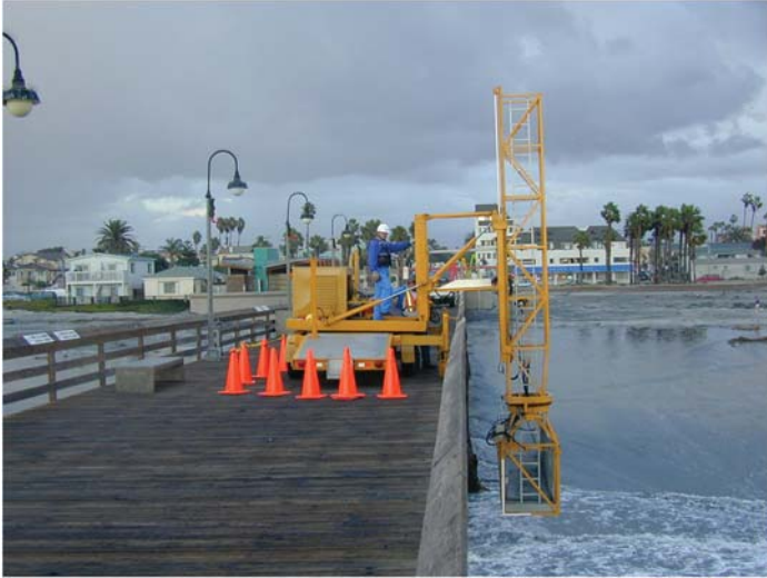
Fig. A-2. Above water inspection team using a man lift to access the underside of a timber pier deck
