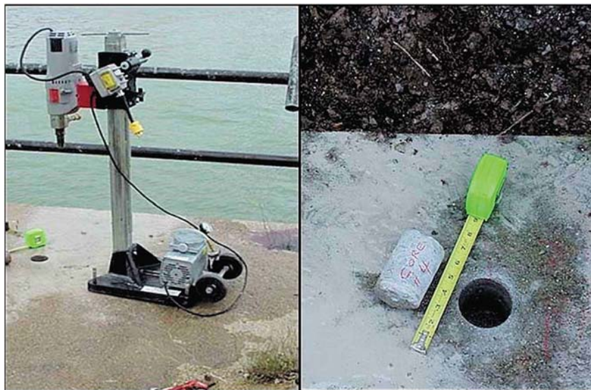
Fig. C-10. Concrete deck core photographs
