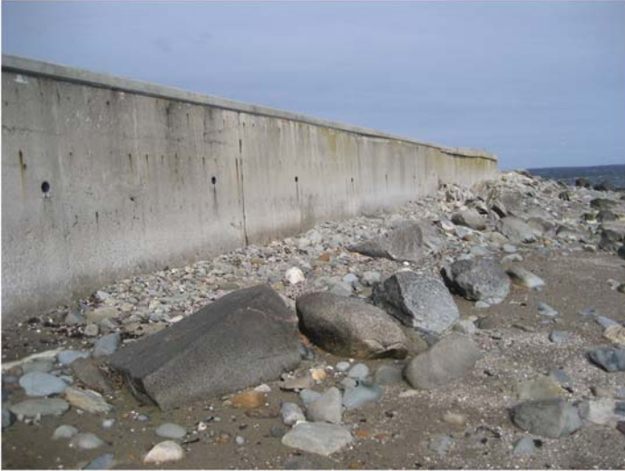
Fig. A-18. Mass concrete seawall
