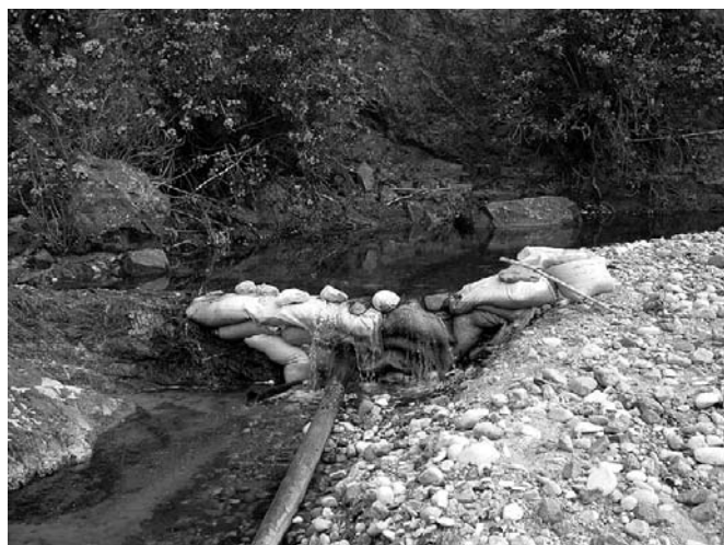
Figure 15.2. Contemporary Bedouin dam in Wadi Ghuwayr, used to help channel water into plastic pipes for transport to fields to west.
