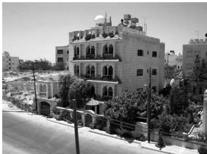
Figure 26.4. Typical roof-top storage tanks on a property in the northwestern suburbs of Amman.
