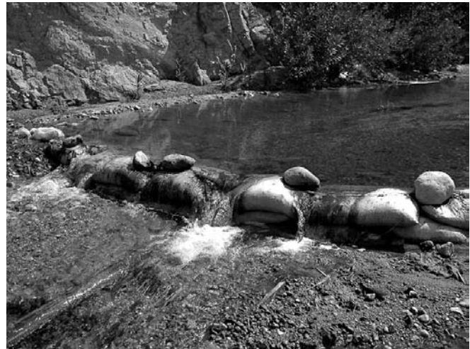
Figure 27.8. Rudimentary dam in Wadi Ghuwayr to collect water prior to transfer through pipes for irrigation.
