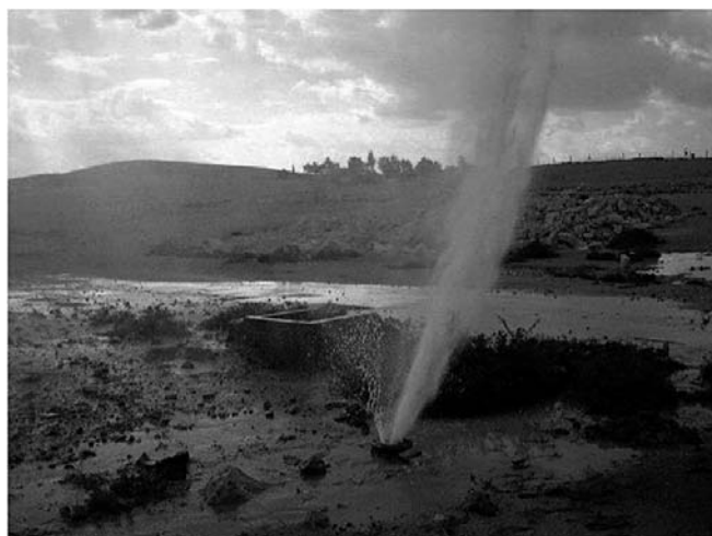
Figure 28.2. An illegal connection from the principal pipe of the network, southern Amman Governorate.
