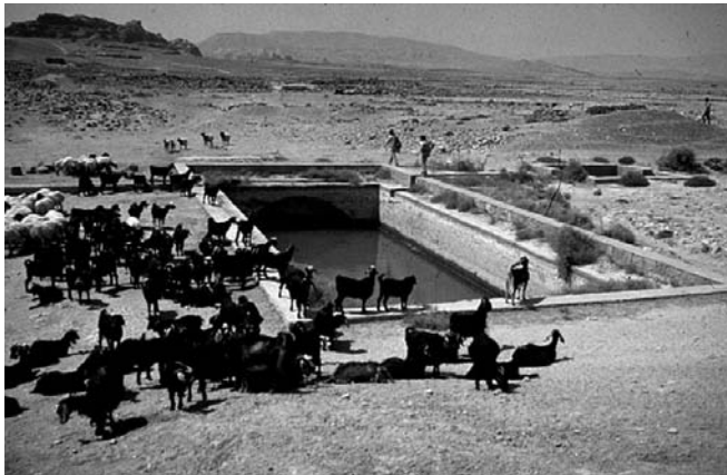
Figure 19.4. Reservoir at Humayma (after modern restoration, originally covered). (Courtesy E. De Bruijn).
