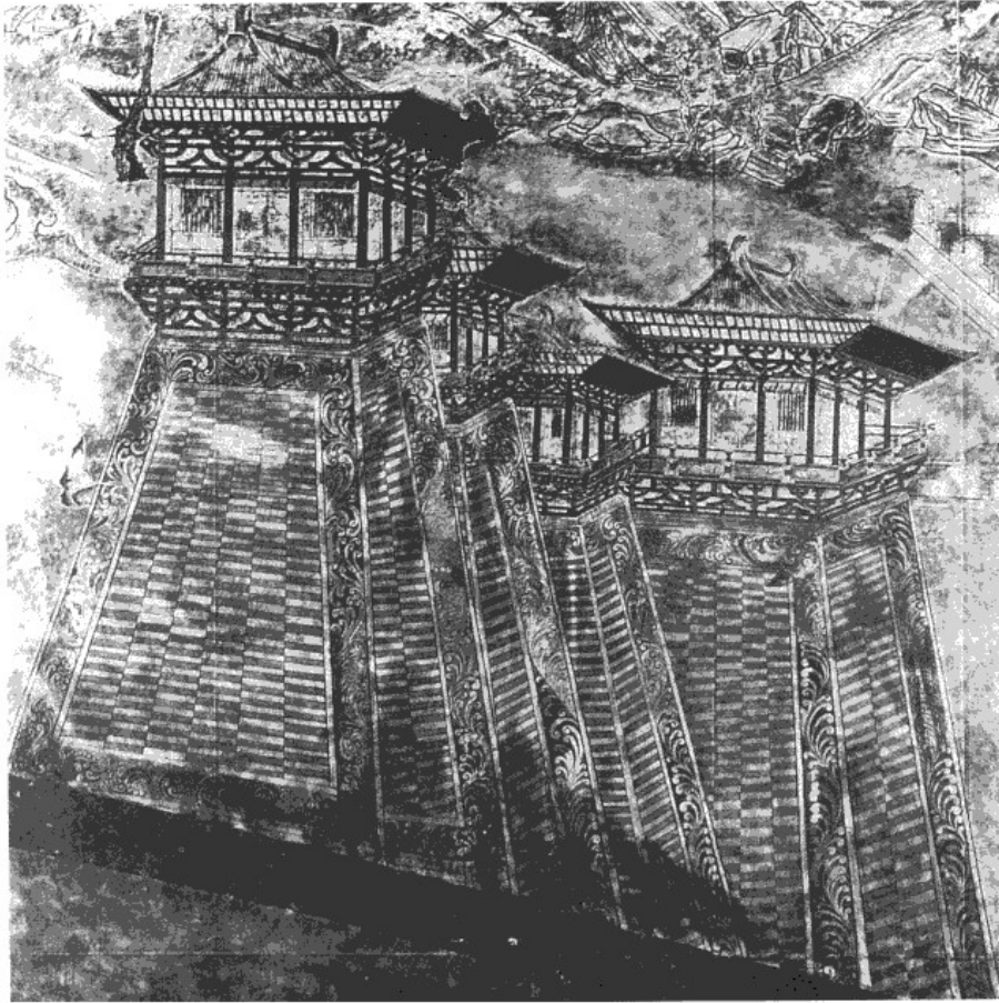
Figure 91. Gate-towers of Chang'an from tomb of Crown Prince Yide (ca. 706), Shaanxi. [ Han-Tang bihua , pl. 86]
