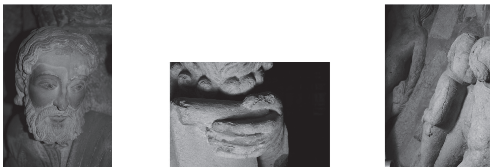
Figure 1. Deterioration processes affecting the Portico de la Gloria, from left to right: efflorescences on the edges of polychromy; arenization due to seritic alteration of the granite; microfractures.
