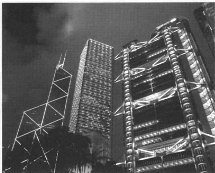
HSBC Headquarters and the Bank of China flanking the Cheung Kong Building.
