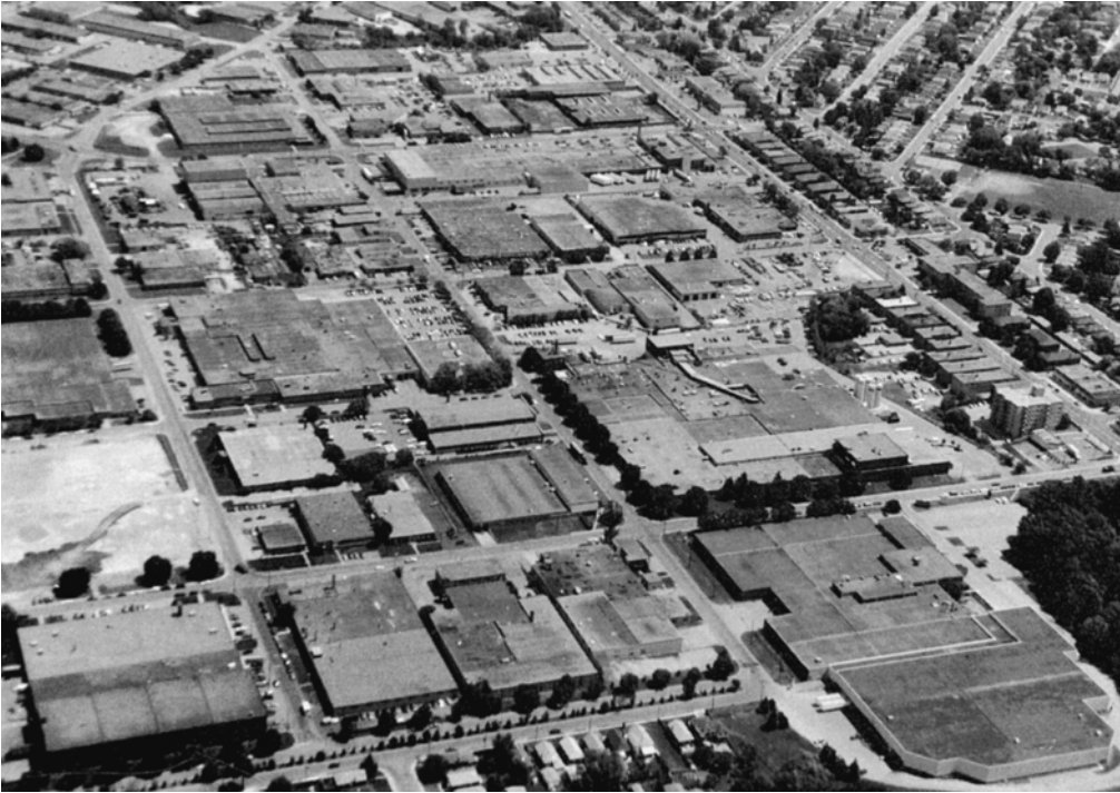
Plate 5.2 Flat rooftops on many industrial buildings offer great opportunities for productive uses, such as gardens, greenhouse production using waste building heat and mini wetlands for wildlife. Compare this North American industrial area with one from Stuttgart, where green roofs have been incorporated into many of the industrial buildings (see Plate 6.8).
