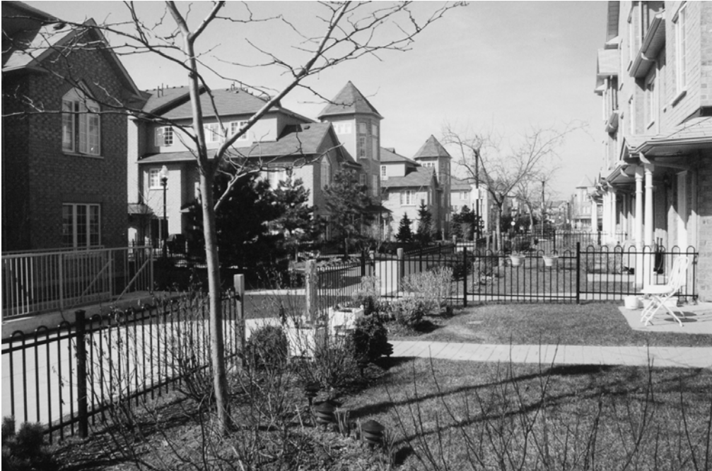
Plate 7.3 Markham Centre, a new urbanism housing development, has responded to the Markham plan respecting Rouge valley edges and sensitive natural features (see colour Plate 3).
