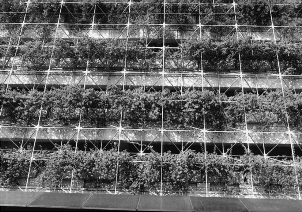
Plate 6.3 Plants covering building walls do more than look nice. In hot climates they can reduce city temperatures by as much as 5°C: a parking garage in Jakarta, Indonesia.
