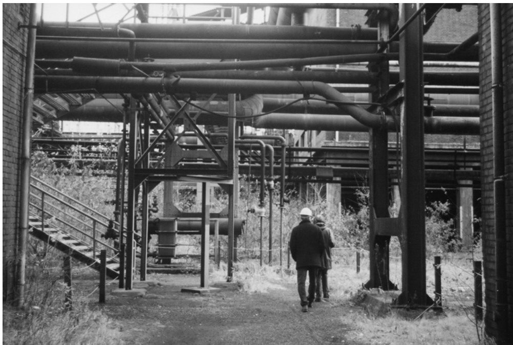
Plate 7.5 The Emscher forests. At ground level, the visual complexity of industrial engineering and emerging vegetation is clearly apparent (see colour Plate 5).
