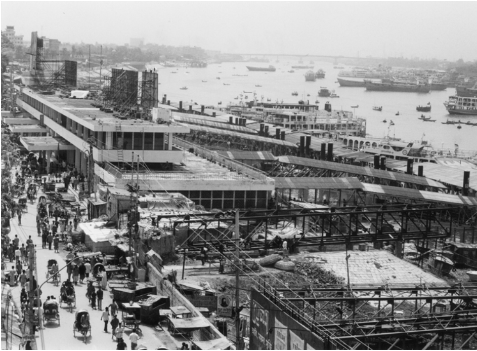
Plate 2.6 A view of the Buckland Bund road where the city first began. The diverse activities in and around this location and its role in linking land and water have made this a distinctive part of the city.
