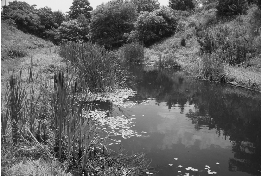
Plate 2.14 Minneola Basin, Long Island. One of the first infiltration basins on Long Island, built in about 1930. It is therefore one of the first in North America. The steep slopes are densely vegetated. In spite of being on the edge of a park, there is no provision for human access other than maintenance.
