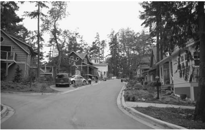
Figure 31-12 Cluster development. As an alternative to conventional subdivisions, this cluster housing development in Port Townsend, Washington, features narrow streets and parking bumpouts instead of garages.
