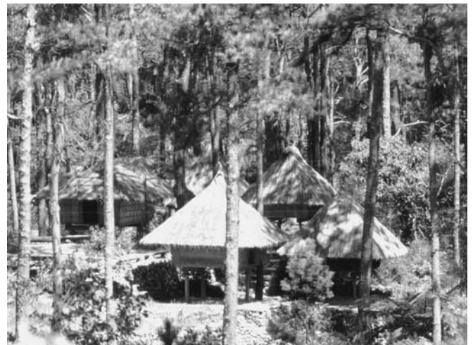
Figure 5-9 Jungle towns in hot-wet climates are constructed less compactly than those in desert climates to avoid blocking cooling breezes. Construction materials such as bamboo and palm leaves are employed to minimize heat retention in buildings (T. Bartuska).
