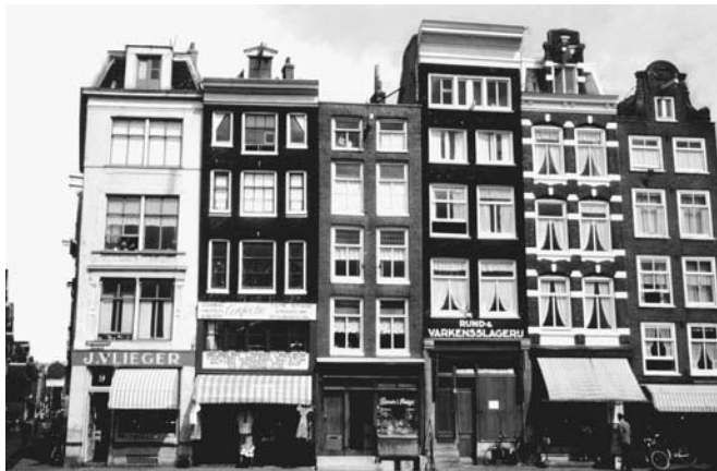
Figure 22-17 Amsterdam today, showing how the 6-meter (20-foot) module is now used (T. Bartuska).
