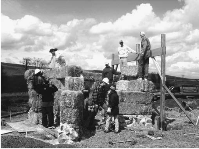
Figure 17-9 Students engaged in a design-build project with straw bale construction (T. Bartuska).
