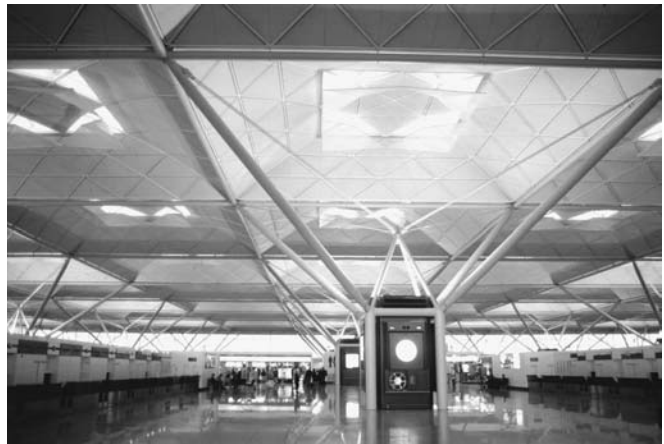
Figure 6-6 An excellent example of systems integration: Stansted Airport by Norman Foster & Associates, north of London, England (T. Bartuska).
