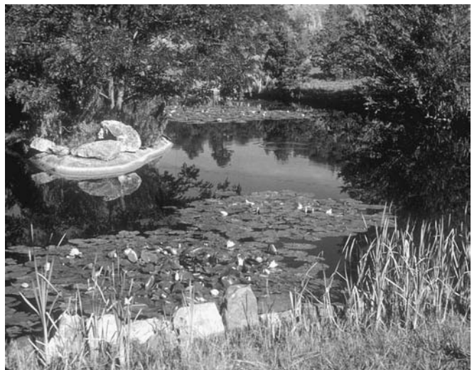
Figure 29-3 The lowest of seven ponds connected by waterfalls at Bishop’s Lodge outside Santa Fe, New Mexico, serves as part of the sewage treatment system for this small resort. Plants help clean the water, which is subsequently used to irrigate adjacent pastures. The owners of the resort use their unique system in their advertising.
