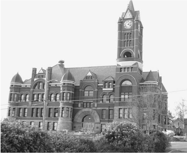
Figure 14-2 Preservation. The Jefferson County Courthouse in Port Townsend, Washington, has been in continuous use as a courthouse since it was constructed in 1892. Repairs continue to be made to keep the building in use without changing its purpose or compromising its historic or architectural integrity. The building serves as an example of ongoing preservation.
