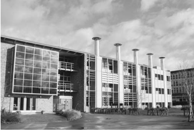
Figure 13-14 A solar-responsive design in which air stacks, chimneys, and operable windows passively ventilate the building. Building Research Establishment (BRE), Watford, England.
