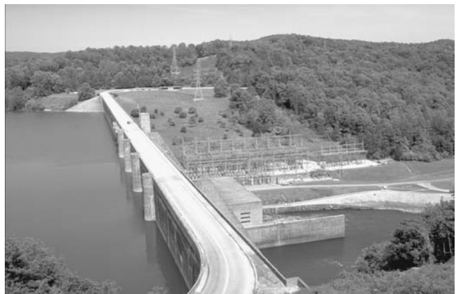
Figure 26-2 Norris Dam was started in 1933 and completed in 1936. It was the first dam built by the TVA. Located in Clinch River in east Tennessee, it is 265 feet high and 1,860 feet long. Its reservoir has a storage capacity of 2.5 million acre-feet of water, of which 1,922,000 is useful, controlled storage. The power installation consists of two 50,400-KW units (courtesy of the Tennessee Valley Authority).
