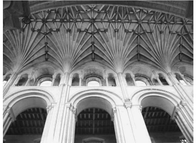
Figure 13-4 Medieval Norwich Cathedral, England—earlier Romanesque round arches (lower level) and later Gothic pointed arches and vaulting (upper level and ceiling).
