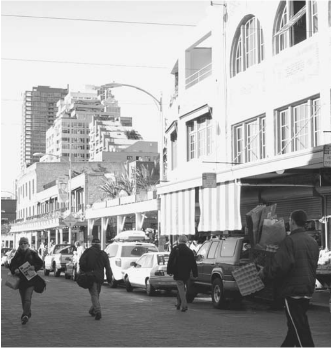
Figure 14-11 Restrictive zoning limiting the height of surrounding development is implemented in the Pike Place Market Historic District to help preserve its intimate street scale.
