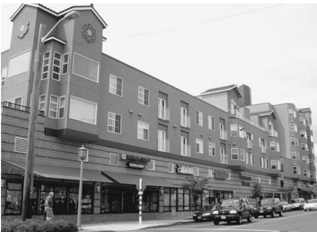
Figure 31-8 Mixed use. A more sustainable concept for a “big box” grocery store in Seattle’s International district. This infill project features housing above and a pedestrian-scale outer layer of retail along the street.
