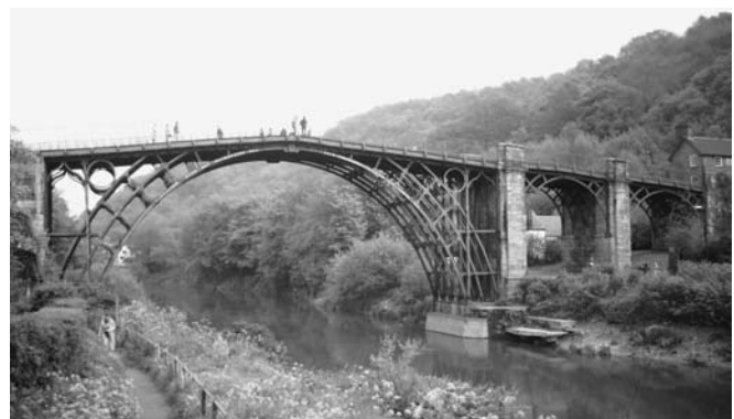
Figure 16-2 The first iron bridge, 1774–1779, Ironbridge, England (T. Bartuska).
