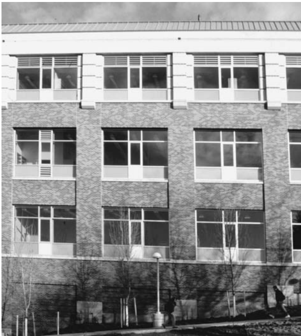
Figures 17-7 and 17-8 A university building during and after construction (T. Bartuska).
