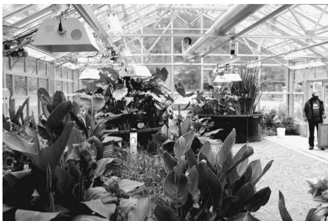
Figure 32-9 Living machine (using plants to process and clean air and water). Islandwood: A School in the Woods, Bainbridge Island, Washington.
