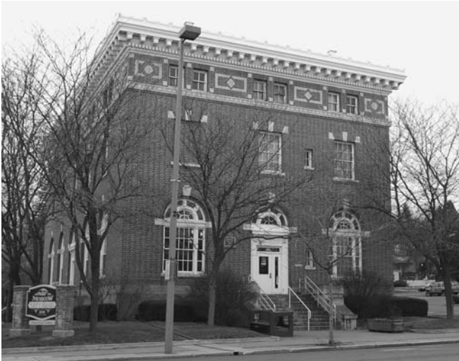
Figure 14-21 Following a twenty-year effort by local citizens and the city, a former 1911 post office in Moscow, Idaho, was adapted to serve as City Hall.
