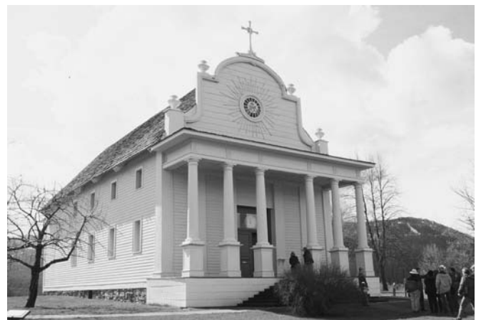
Figure 14-3 Restoration. Constructed in 1865 by French missionary Father Ravalli and members of the Coeur d’Alene (Schitsu’umsh) tribe, Cataldo Mission is the oldest surviving building in Idaho. The mission represents the use of restoration as a preservation strategy.
