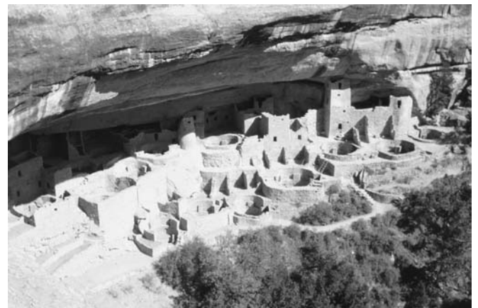
Figure 2-6 Cliff dwellings of the Anasazi Indians at Mesa Verde, Colorado. Heavy masonry walls absorb the heat of the low winter sun, while the overhanging cliff provides protection from the high summer sun.
