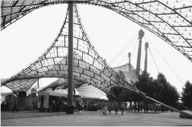
Figure 6-5 A spiderweb network of tension structures by Frei Otto, 1972, Munich, Germany (T. Bartuska).
