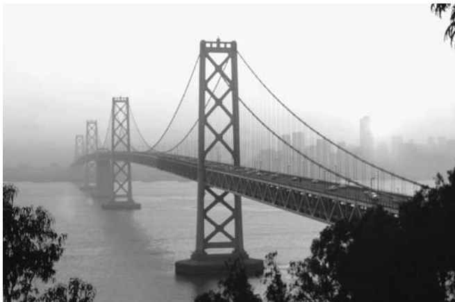
Figure 6-2 A structure that connects two points using “legs” (steel members) and “tendons” (cables) for support: the San Francisco–Oakland Bay Bridge, San Francisco, California (T. Bartuska).
