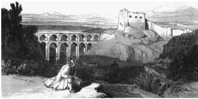
Figure 2-1 Systems of water supply and defense, a Roman aqueduct and a medieval castle, dominate a landscape. Arghyrokastrò, Albania (E. Lear, 1848).
