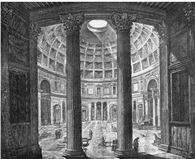
Figure 2-16 The Pantheon, Rome, 120 C.E. A vast interior space relying on sheer mass for stability. The only opening is the oculus at the top.
