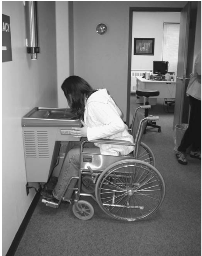
Figure 4-4 Accessible drinking fountain (Pamela Overholtzer).
