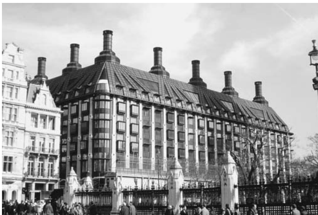
Figure 13-15 Air stack-chimneys, and operable windows that passively ventilate the building. New Parliament Building, London, England (architect, Hopkins).
