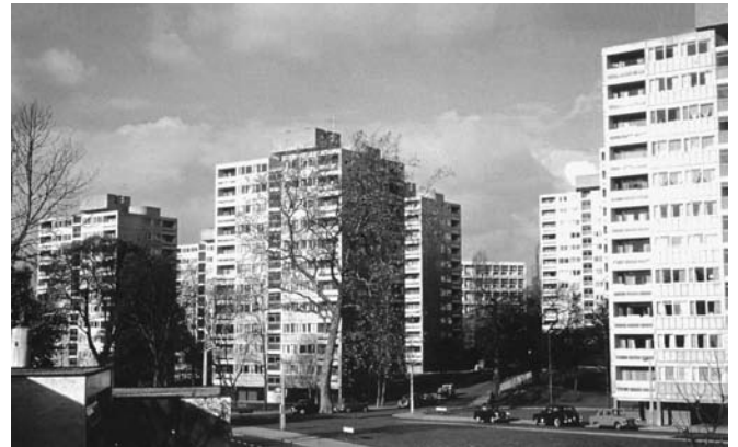
Figure 2-21 High-rise housing at Roehampton, near London, built in the 1950s. An award-winning project that was later criticized for being unsuited to family life.
