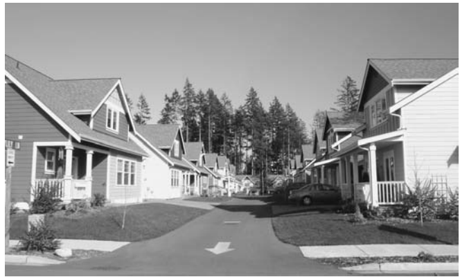
Figures 17-2 and 17-3 Residential townhouse and cottage housing during and after construction (T. Bartuska).
