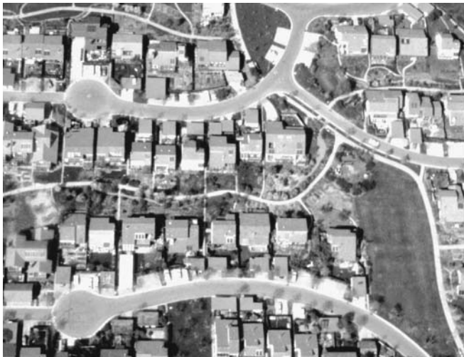
Figure 23-5 Subdivision patterns of walkways and streets. Village Houses, Davis, California (courtesy of Sandra Satterlee).
