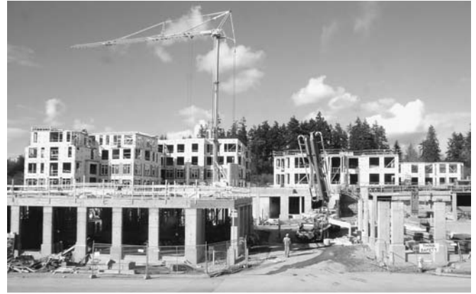
Figure 17-10 Mixed-use housing project: commercial and parking base with townhouses and apartments above (T. Bartuska).
