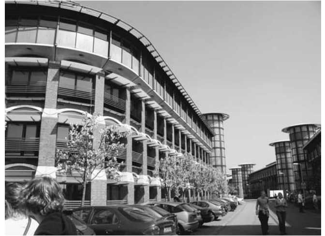
Figure 13-16 Effective window shading, daylight strategies, air stacks, chimneys, and operable windows that passively ventilate the building. Inland Revenue Complex, Nottingham, England (architect, Hopkins).
