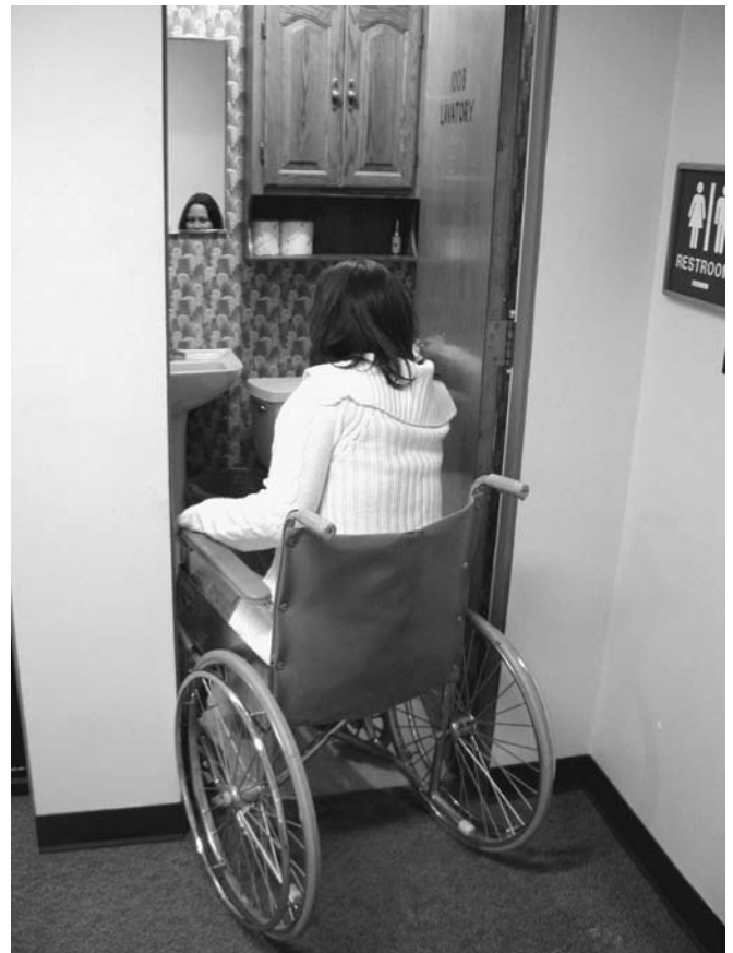
Figure 4-2 Accessibility. The built environment must accommodate individuals with disabilities. The photo illustrates the restriction to free access that a wheelchair-bound woman encounters as she tries to use the restroom because the doorway is too narrow (Pamela Overholtzer).
