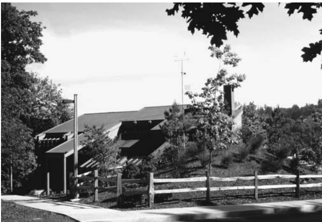
Figures 15-11 and 15-12 Solar demonstration home, Portland, Oregon. Warm south side, cool north side.
