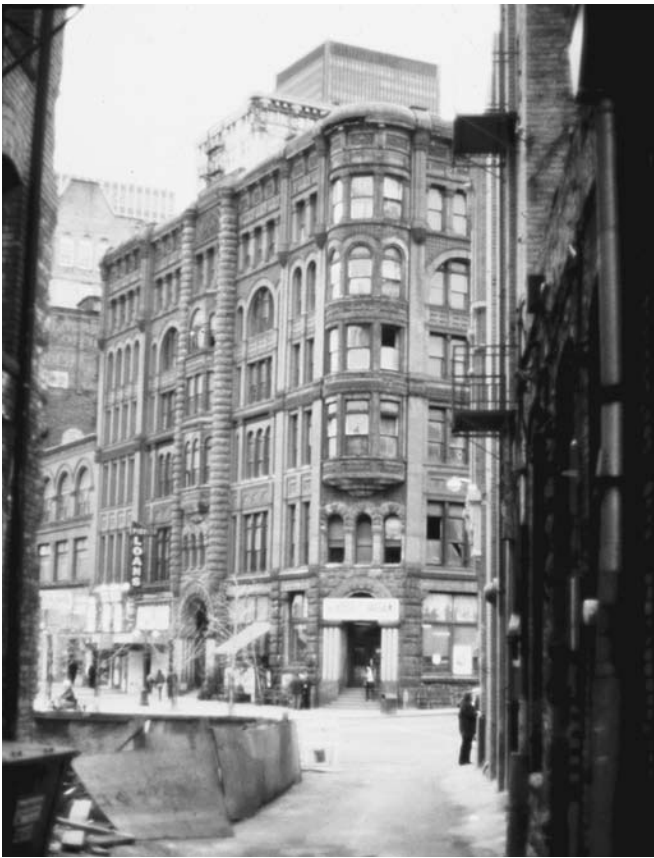
Figure 14-13 Before—photo taken by visionary architect Ralph Anderson of the Pioneer Building in Seattle on Pioneer Square demonstrates the condition of buildings in the district before they were rehabilitated.
