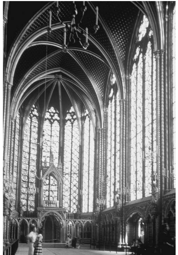
Figure 10-1 Ste. Chappelle is an excellent example of Gothic construction. Notice the emphasis on height and the large number of windows relative to the structure (Patrick Snadon).
