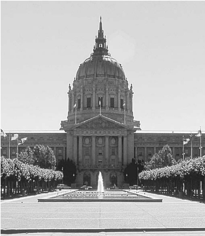
Figure 20-4 San Francisco's City Hall campus.
