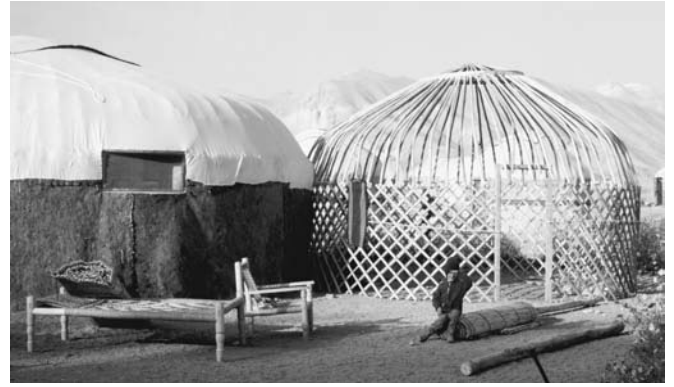
Figure 2-5 The yurt is ideally adapted to the life of nomads in Afghanistan. It collapses for transportation, yet provides protection in a harsh climate (T. Bartuska).
