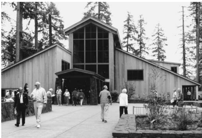
Figure 12-11 The Americans with Disabilities Act helps ensure a barrier-free public built environment. This picture shows the level entry of the Mount Saint Helens Visitors Center in Washington.
