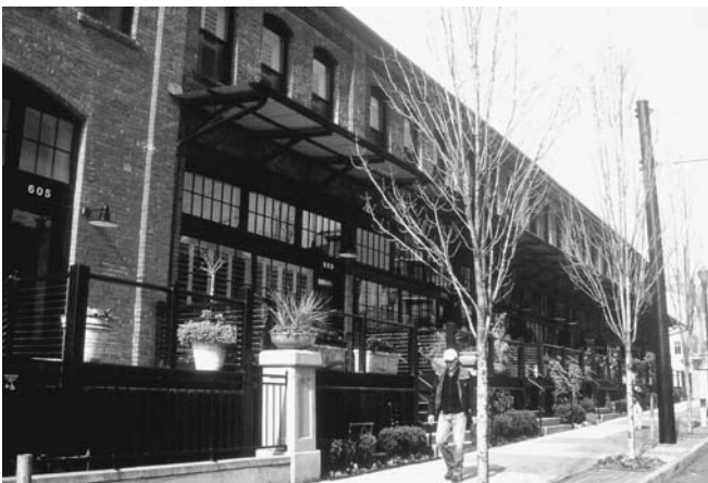
Figure 31-4 Adaptive use. The ultimate recycling program. Embodied energy in this former warehouse in the historic Pearl District of Portland, Oregon, is captured with conversion of the structure to luxury condominiums to “warehouse” people.
