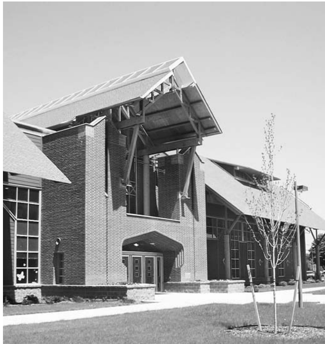
Figure 29-5 The new Recreation Center on the University of Idaho campus uses manufactured wood products to form the roof trusses that emphasize the entry to the building. Designers used a wide variety of resource-efficient materials throughout the structure. Students were also deeply involved in setting the design agenda for their building, and its central location encourages pedestrian accessibility and minimizes the use of automobiles.
