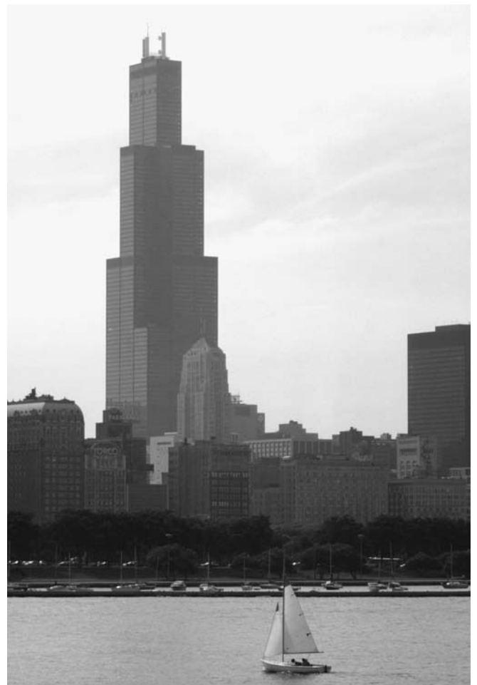
Figure 6-7 One of the world's tallest buildings: The 109-story Sears Tower by Skidmore, Owings & Merrill, 1974, Chicago, Illinois (T. Bartuska).
