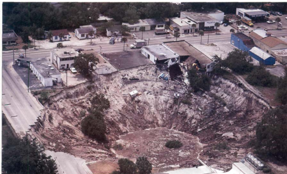
Figure 11.17 Most of a city block in Winter Park, Florida disappeared into a widening crater as this sinkhole formed in underlying carbonate bedrock.
