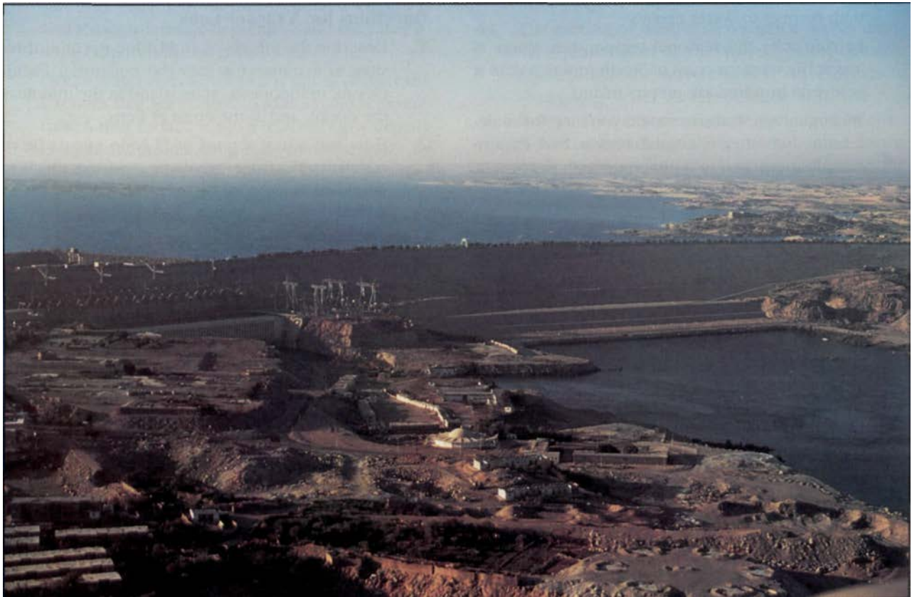
View of Aswan High Dam, which impounds the Nile River (right) to form Lake Nasser impounds (to south, behind dam). Sediment formerly carried northward to the Mediterranean Sea and now settling out in the lake will eventually fill the reservoir and make it unusable.
