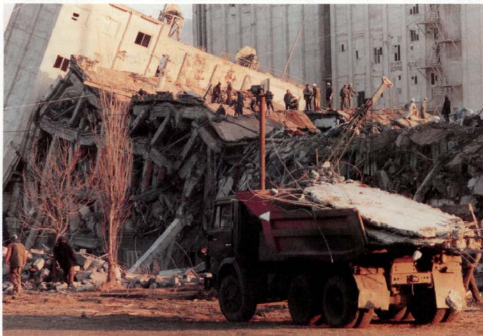
Figure 3.11 When a magnitude 6.8 earthquake struck Armenia on December 7, 1988, poorly constructed buildings with inadequate foundations collapsed like houses of cards. The principal cause of collapse was ground motion.
