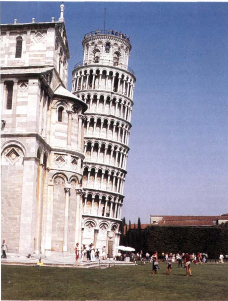
Figure 9.26 The Leaning Tower of Pisa, Italy, the tilting of which accelerated as groundwater was withdrawn from aquifers to supply the growing city.
