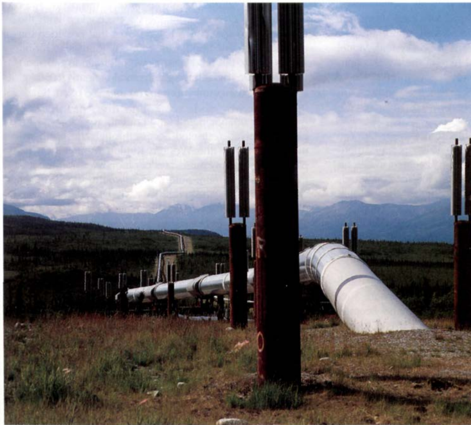
Figure 10.24 The Alaska Pipeline carries petroleum from the North Slope oil fields near Prudoe Bay southward across two mountain ranges enroute to the port of Valdez. To increase the ease of flow through the pipe, the oil is heated. Because much of the pipeline route lies across permafrost terrain, in many sectors the huge pipe is suspended above ground on large piers to keep it from melting the frozen ground beneath.
