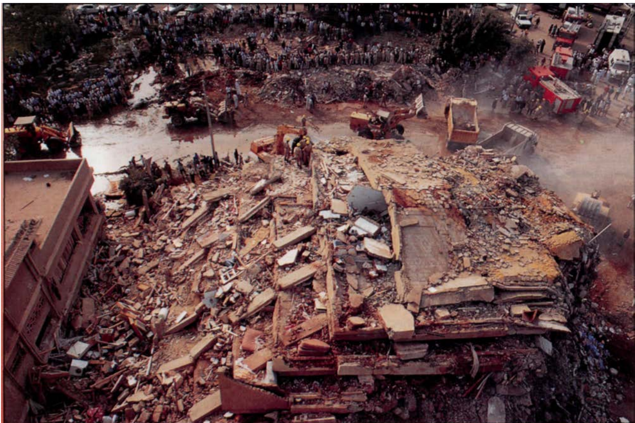
Damage in Cairo, Egypt, caused by an earthquake, magnitude 5.9, on October 12, 1992. Several factors accounted for the severity of damage: the earthquake focus was at a depth of 10 km immediately below Cairo. The city is densely populated, many dwellings are not built to withstand earthquakes, and much of the city is built on weak, unconsolidated sediment deposited by the River Nile.
