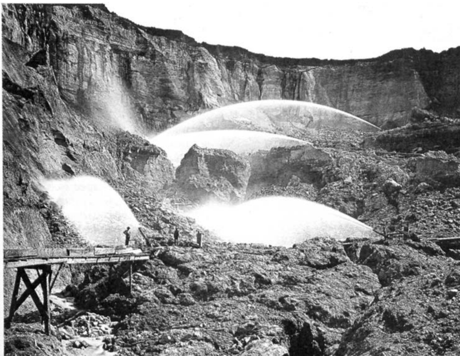
Figure 9.25 Hydraulic mining in the foothills of California's Sierra Nevada. Gold-bearing alluvium is washed into wooden channels (sluices) where flakes and nuggets of gold are concentrated. Although this was an efficient way of mining in the years following the Gold Rush, it led to widespread environmental degradation of streams, and its impact was felt as far away as San Francisco Bay.
