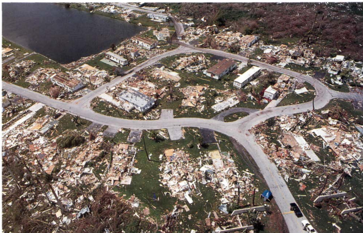
Figure 13.1 All that remains of a town in Florida after Hurricane Andrew passed through in 1992. All the damage seen here was caused by high speed winds.
