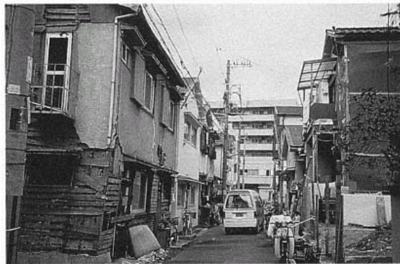
Figure 65 Patched-Over Damage along Narrow Street. In residential areas with partial damage, the "standards of repair" have been determined by individual owners. Blue plastic tarps are a common sight. (Charles Eadie)
