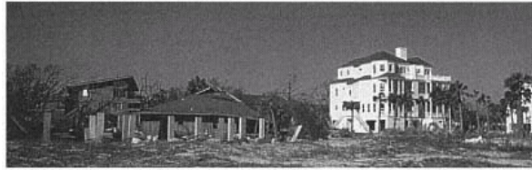
Figure 10 Houses, 57th Avenue, Isle of Palms. The house on the right suffered considerably less damage than the one on the left because it had been elevated to protect it against storm surge. (Peter R. Sparks)
