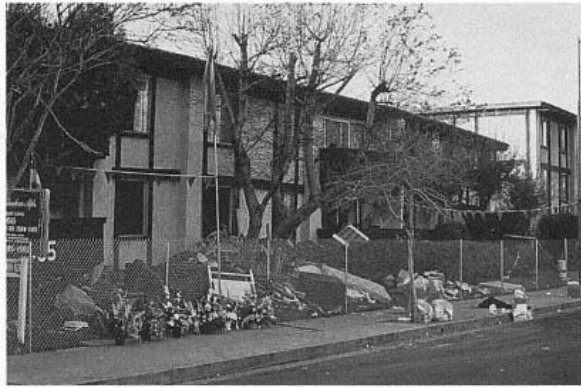
Figure 36 Collapse of Northridge Meadows Apartment Building. Sixteen people died in the collapse. (© J. Scott Smith)
