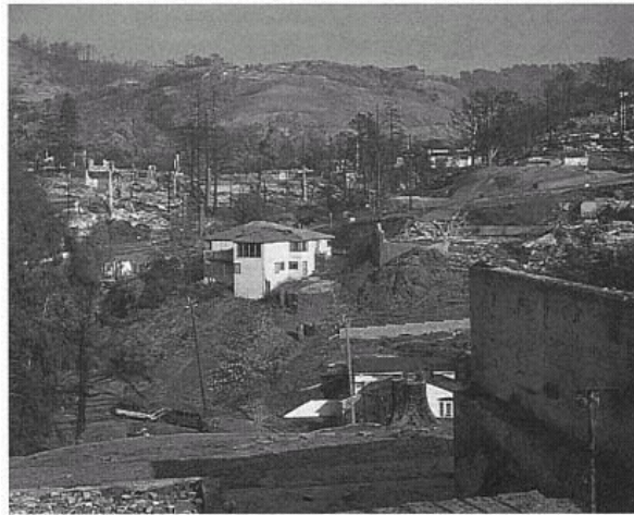
Figure 46 Single House Remaining after 1991 Oakland Hills Fire. Few houses survived the intense heat and flames that devastated three thousand homes in the Oakland and Berkeley Hills. (California Governor's Office of Emergency Services, Earthquake Program)
