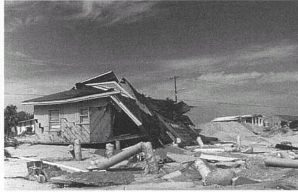
Figure 9 Beach House, Garden City, South Carolina. Beachfront properties were damaged by a combination of erosion, floodwaters, and wind. (Peter R. Sparks)
