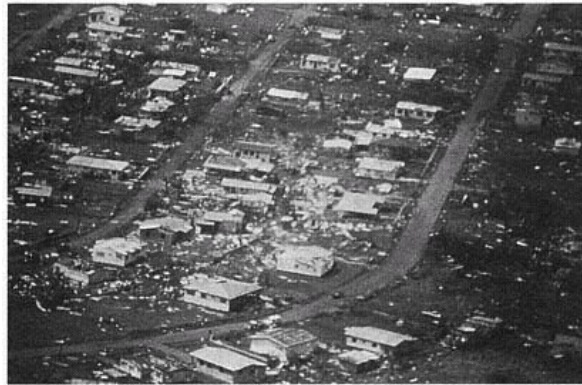
Figure 15 Aerial View of Damage to Moderate-Income Housing. Poorly built inland housing suffered damage similar to that of beachfront properties. (National Oceanic and Atmospheric Administration Photo Library)
