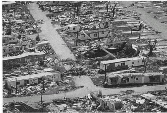
Figure 30 Aerial View of Damage to Manufactured Homes. A mobile home park near Harris Field in Homestead was devastated by the storm. (© The Miami Herald /David Walters)
