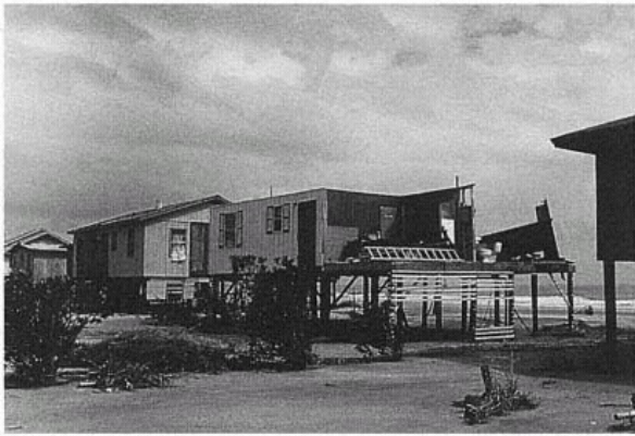
Figure 1 Housing Damage, Hurricane Hugo. Hurricane damage to residential structures is caused by high wind and storm surge. (Peter R. Sparks)
