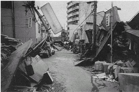
Figure 58 Narrow Street with Buildings Fallen, Kobe. Many concrete buildings collapsed from damage to first-floor columns. (Laurence Kornfield, City of San Francisco)
