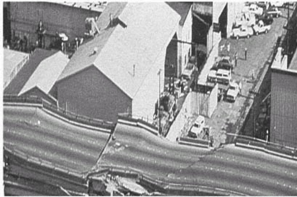
Figure 18 Aerial View of Cypress Freeway Collapse. A 1.6-kilometer segment of double-deck freeway collapsed in West Oakland. (Earthquake Engineering Research Institute's slide collection)
