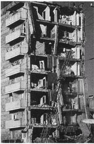
Figure 47 Housing Damage in the Armenian Earthquake, 1988. Damage to concrete-frame buildings with masonry infill walls was extensive. (California Governor's Office of Emergency Services, Earthquake Program)
