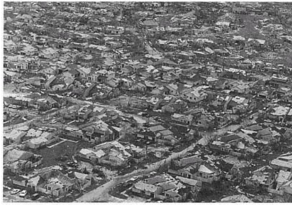
Figure 28 Aerial View of Country Walk Area of South Dade County. Here, nearly all homes suffered some damage and many were completely destroyed. (© The Miami Herald /Joe Rimkus Jr.)
