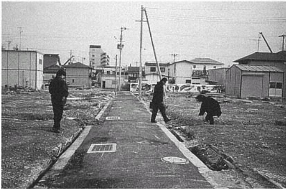
Figure 60 Nagata Ward after Fire. Narrow streets are all that remain of the densely built area. (Catherine Bauman)
