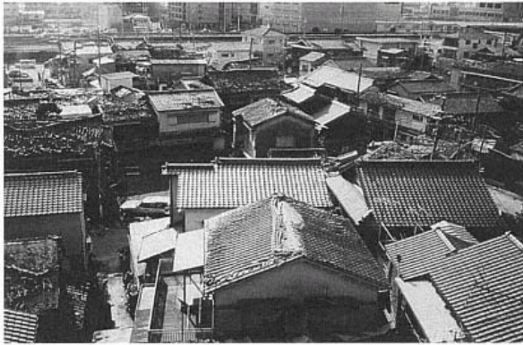
Figure 59 Damaged Tile Roofs. Heavy tiled roofs, designed as storm protection, collapsed killing thousands of sleeping residents. (Catherine Bauman)
