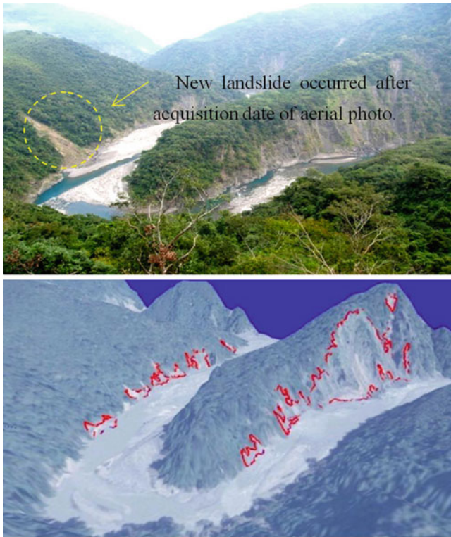
Fig. 6.10 Comparison between global detection results and on-site surveying
