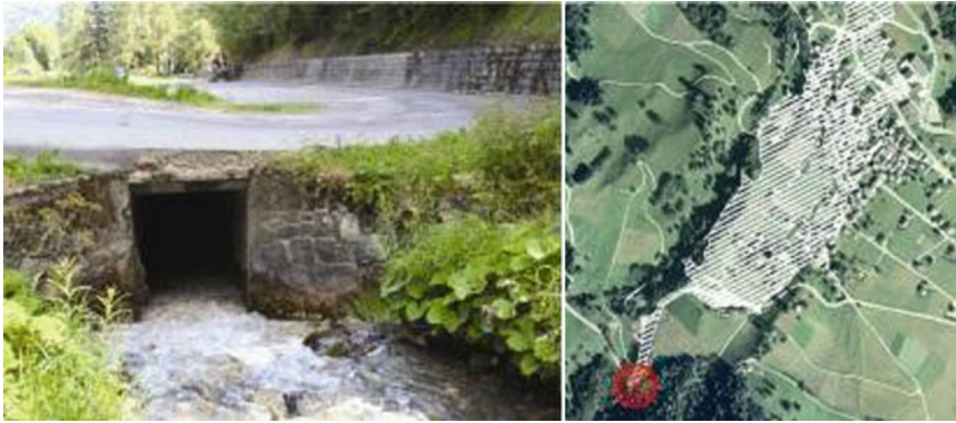
Fig. 5.28 An example of a potential source of overflow and its corresponding modeled spreading (orthophoto: ©swisstopo)
