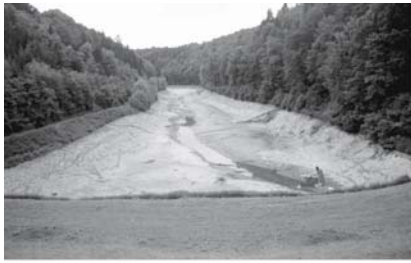
Flood retention reservoir: deposited sediments
