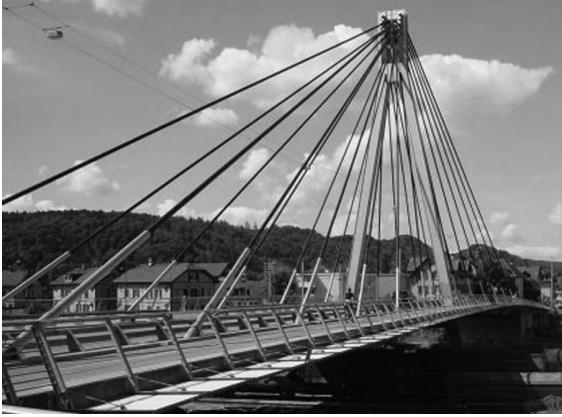
174 Stork Bridge, Winterthur, Switzerland. (Source: Used with permission from Reference 39.)
