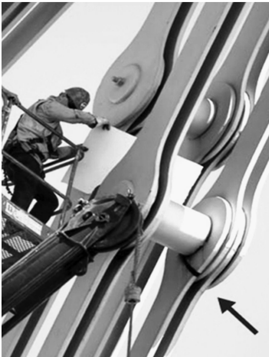
6.9 Crack location. 30
