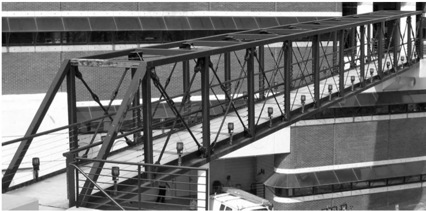
15.15 Picture of the space frame bridge on Georgia Tech campus.
