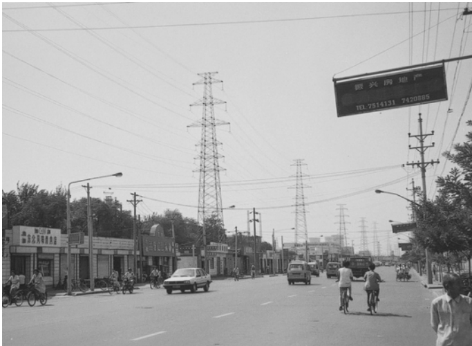
Plate 22 Power lines emanating from the Zhengzhou Heat and Power Plant (Henan)
