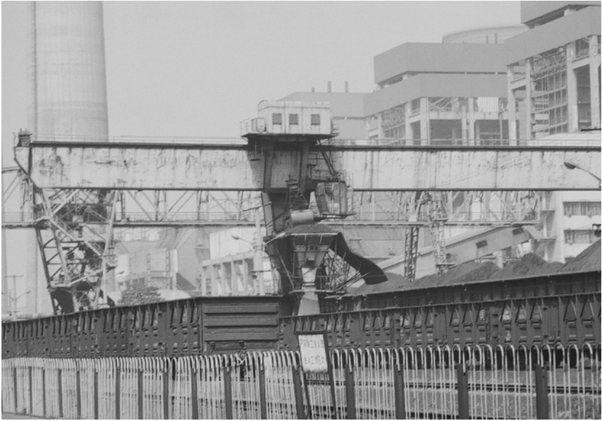
Plate 9 Railway cars loaded mechanically in Zhengzhou (Henan)
