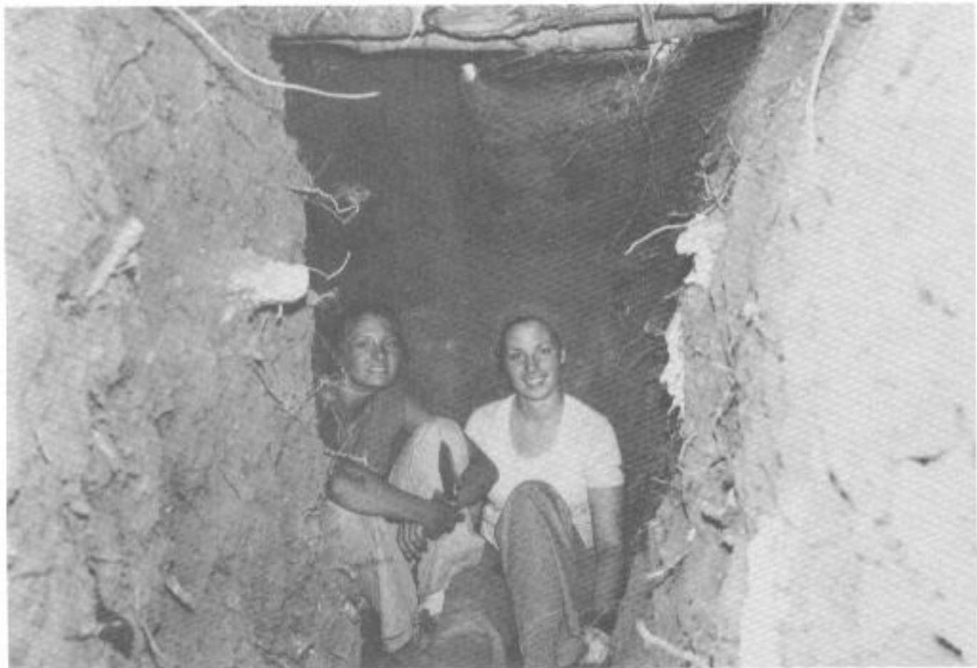
Fig. 5.2. Two non-athletic college girls who completed a 4-person Pole-Covered Trench Shelter in 35 \frac{1}{2} hours, despite tree roots.
