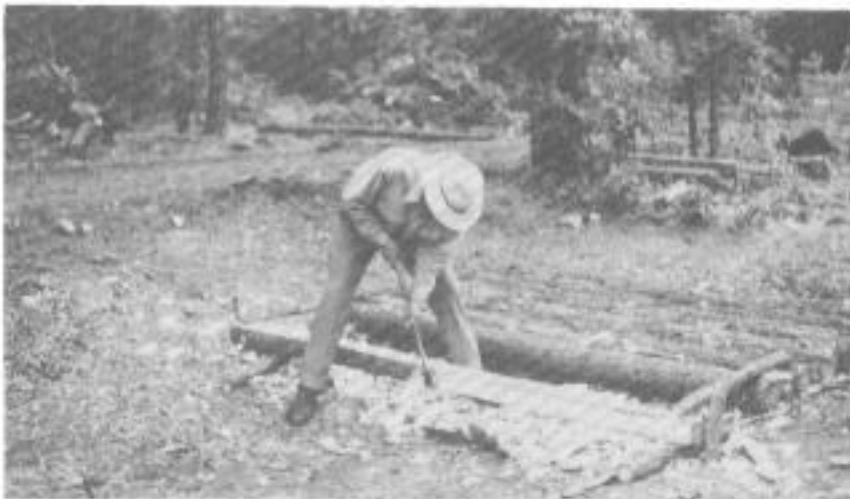
Fig. D.17. Hewing flat sides on a pole with a sharp ax.
