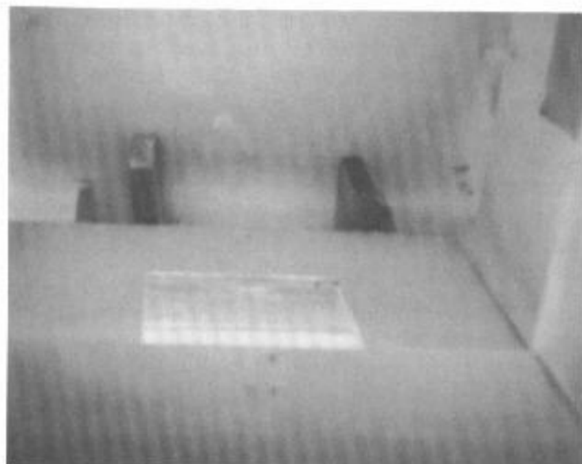
Fig. F.4. View from Below the Exit, Looking Up the Multi-Purpose Emergency Exit Housing. The top is shown supported in a tilted position by two 6-inch-wide boards placed between a wall and the top.
