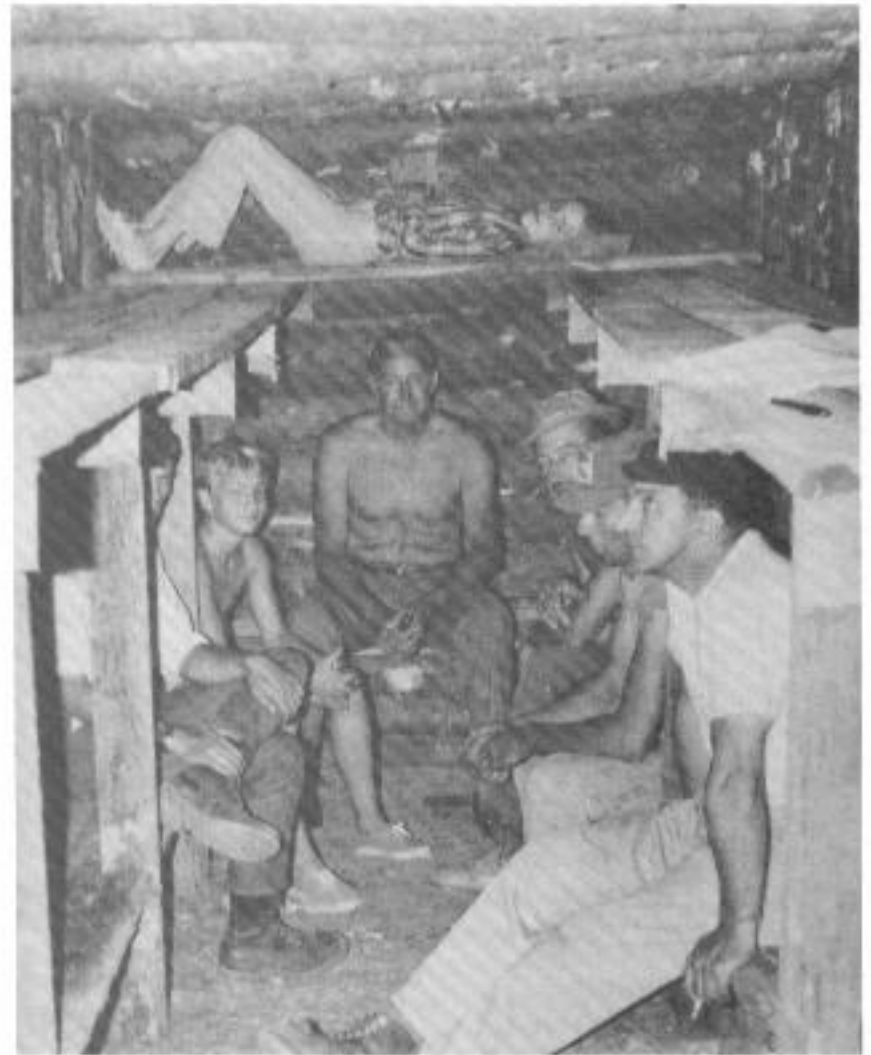
Fig. 14.2. Benches with overhead bunks in a skillfully designed Small-Pole Shelter of Russian design. Three rural families in a wooded area of Tennessee built this expedient blast shelter in 48 hours, including the time spent felling trees and making furnishings.
