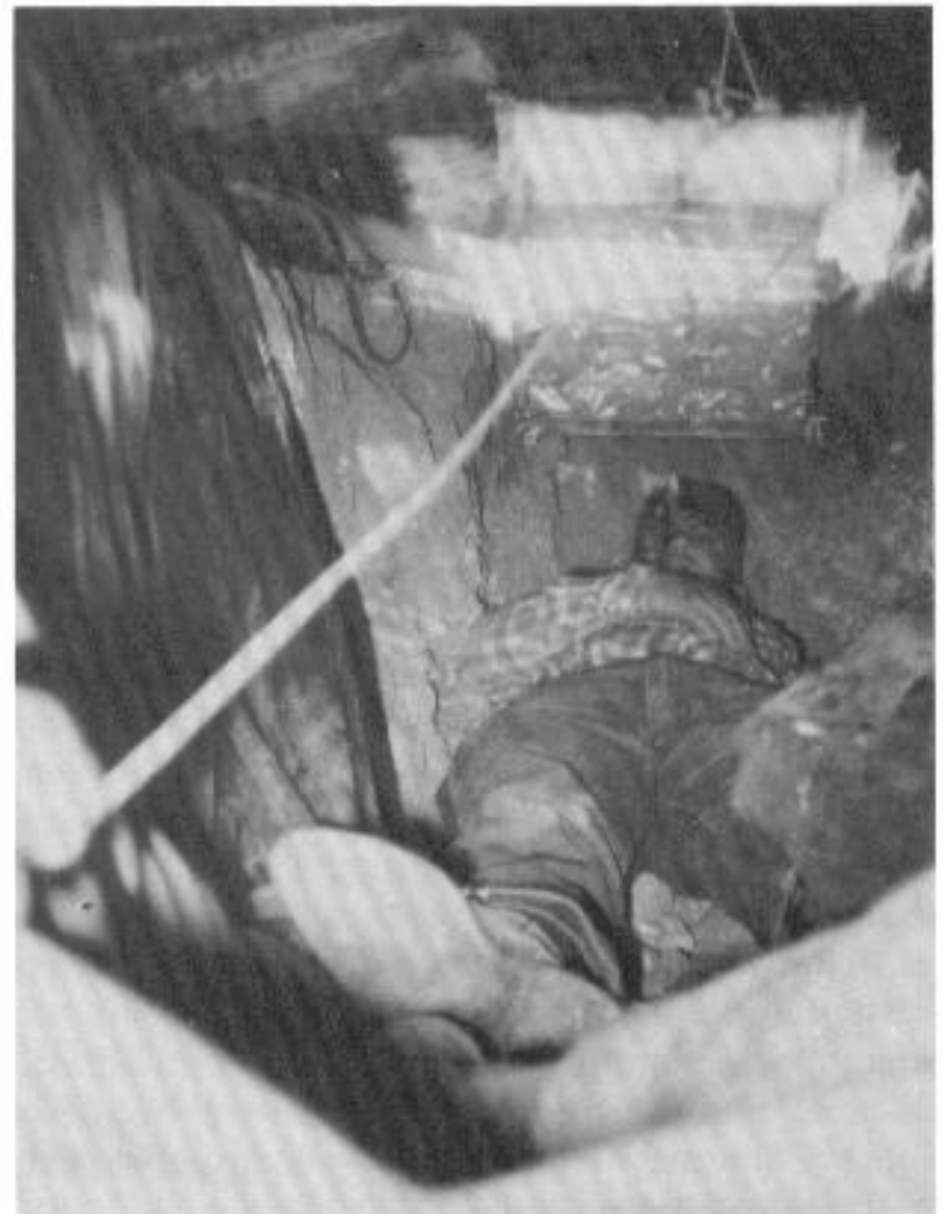
Fig. 6.3. Pulling a Small, Stick-Frame KAP to Keep Temperatures Endurable for Occupants of a Car-Over-Trench Shelter in Warm Weather. Enough air also can be supplied with a small Directional Fan, although more laboriously.
