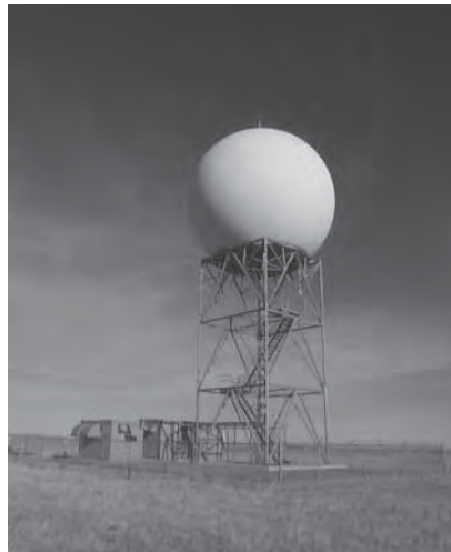
FIGURE 19.2 Nexrad WSR-88D radar at Missoula, Montana, mounted on 15-m tower with two equipment shelters—one containing the transmitter, receiver, processor, and communications equipment, and the other containing a standby generator (Photo courtesy of NOAA/NWS)
