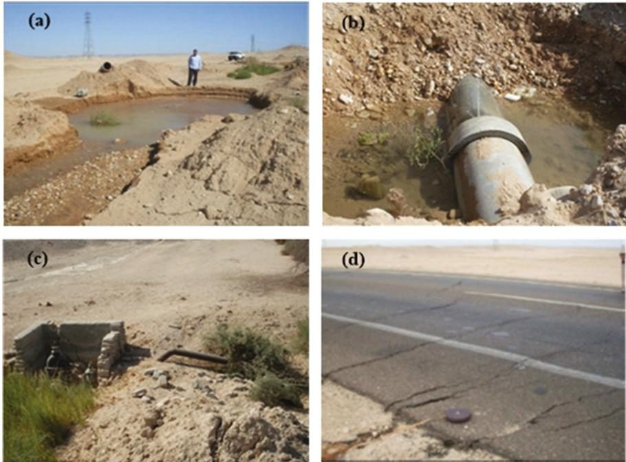
**Fig. 2.** Some examples of the damages caused by the fractures on the sides of Qena-Safaga Road. In (a), (b) and (c), the fractures damaged the buried water pipes that run parallel to the road. (d) shows cracking of the main asphalt road by the fractures (after Galal 2012)
