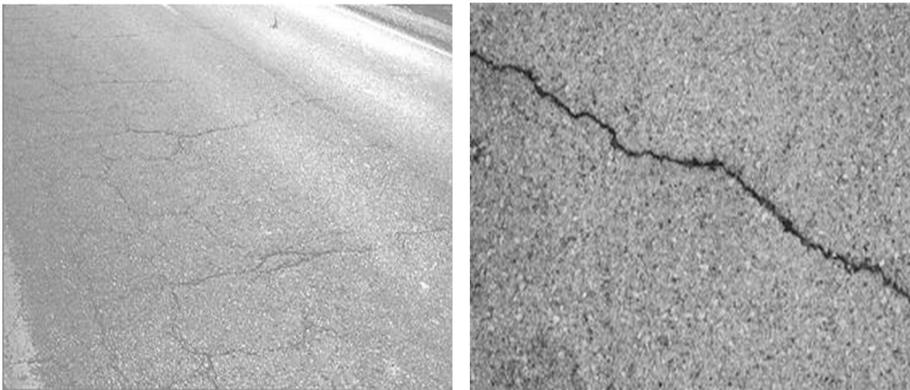
**Fig. 2.** A site photograph of a fractured road founded on an expansive clay bed in the studied area
