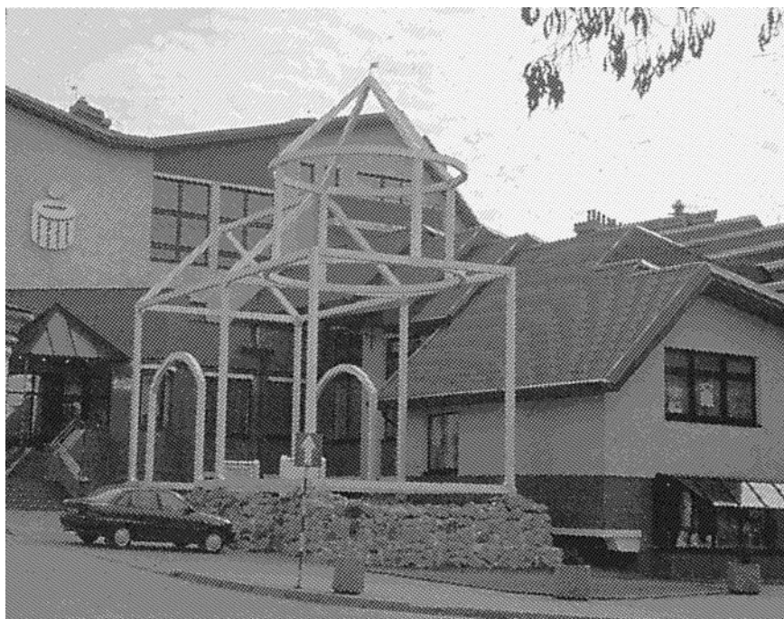
FIGURE 3. Medieval gate building at Ostróda in the north-eastern Poland reconstructed in the form of a structural phantom after archaeological excavation. Phot. Z. Kobyliński
