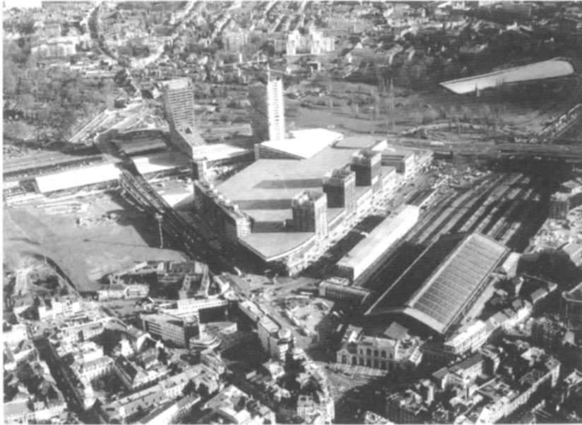
Fig. 5.3 Euralille, the place. Lille-Flandres is at the bottom right of the picture, Lille-Europe at the top left. The city centre is at the bottom; peripheral residential neighbourhoods are at the top. Between the two stations is the new multifunctional complex of Euralille. Just outside the picture, at the top right, is the new event, congress and exhibition centre. (Source: Euralille. Photo: NAI)
