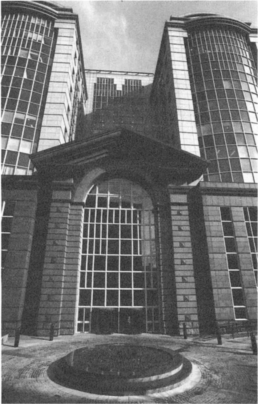
Plate 6 Beaufort House, Aldgate
