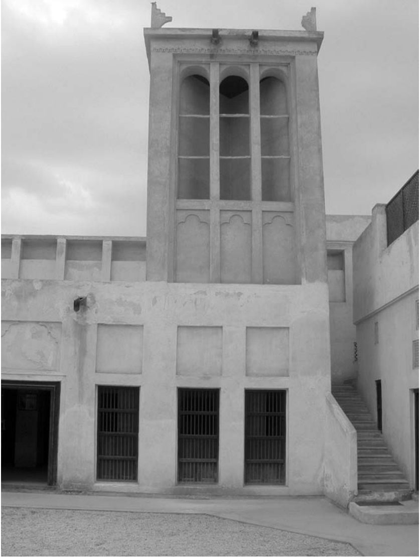
Fig. 1 Sheikh Isa Bey House Bahrain: wind tower above reception room.
