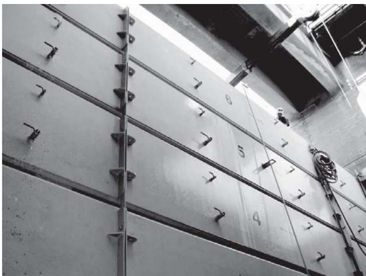
**Figure 2-24. Articulated floating bulkhead, installed.**
