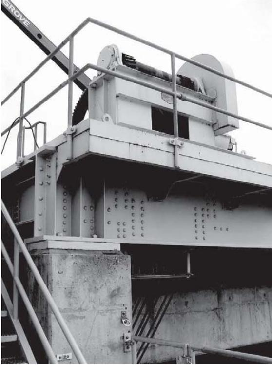
Figure 2-63. Multiple Rope Hoist.
