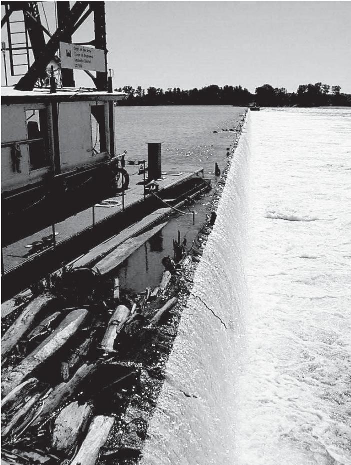
Figure 2-19. Wicket gates (manual placement type)
