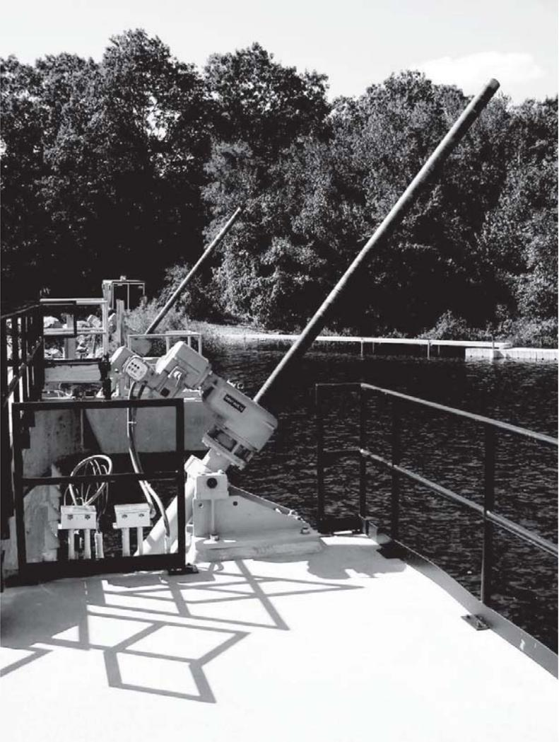
Figure 2-69. Screw stem gate operator.
