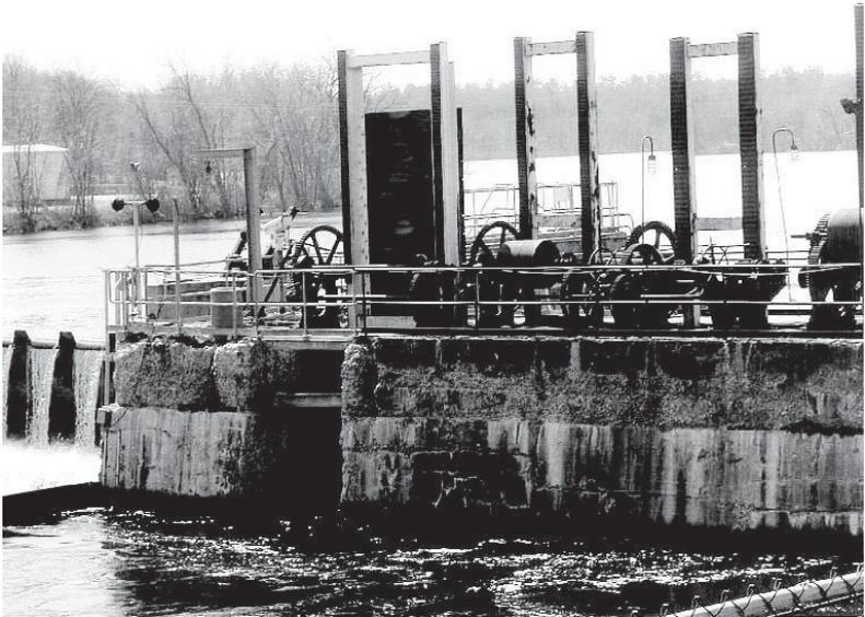
Figure 2-68. Rack and pinion gate operator.
