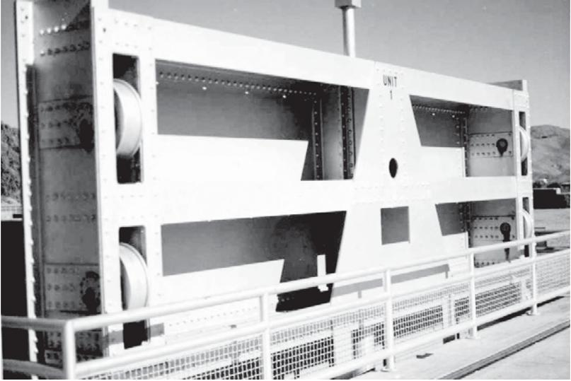
Figure 2-35. Wheel-mounted gate (Courtesy of USBR).
