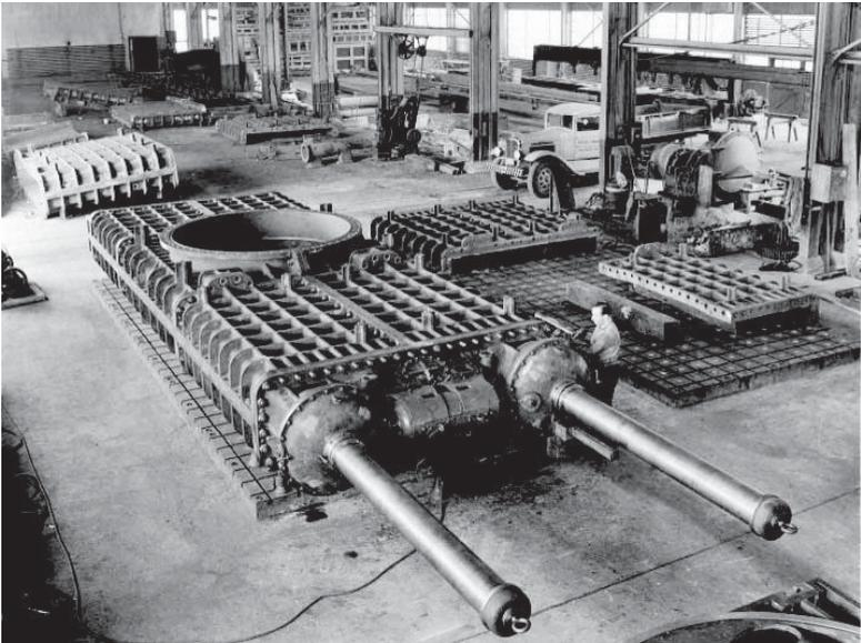
Figure 2-38. Paradox gate (Courtesy of USBR).
