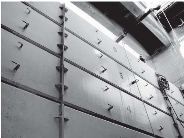
Figure 2-24. Articulated floating bulkhead, installed.
