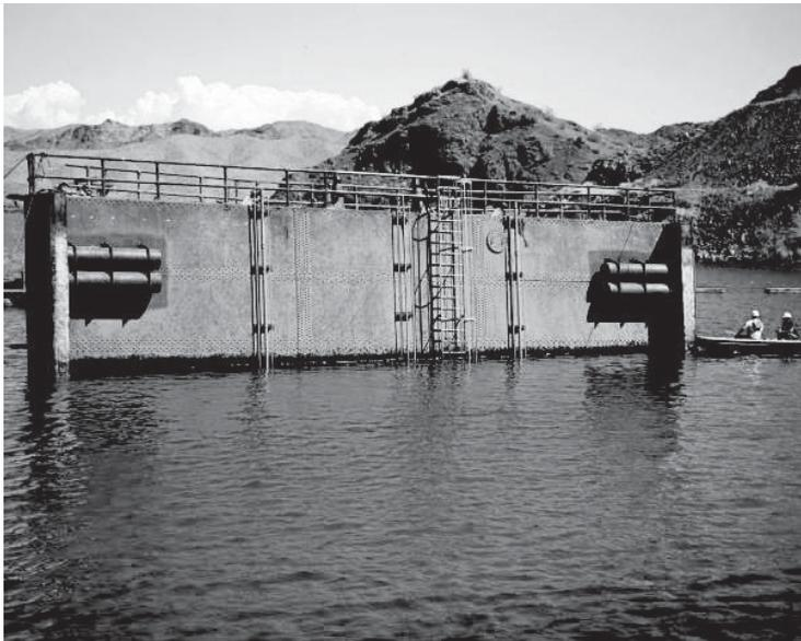
Figure 2-23. Single-piece floating bulkhead being positioned.
