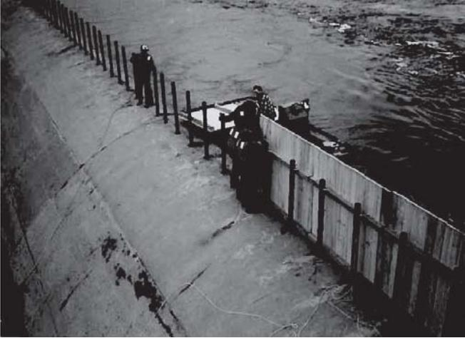
Figure 2-13. Installation of pinned flashboards.
