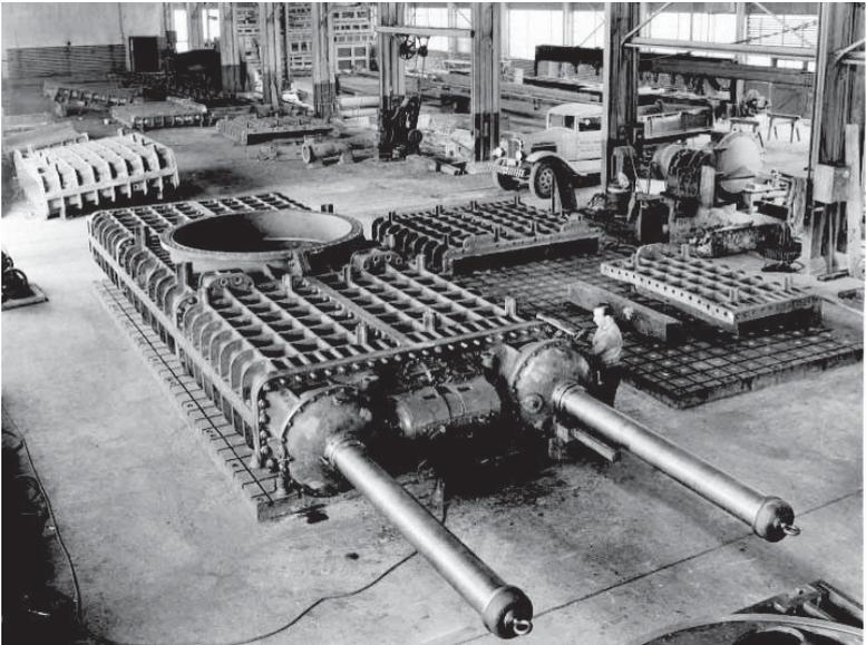
Figure 2-38. Paradox gate (Courtesy of USBR).
