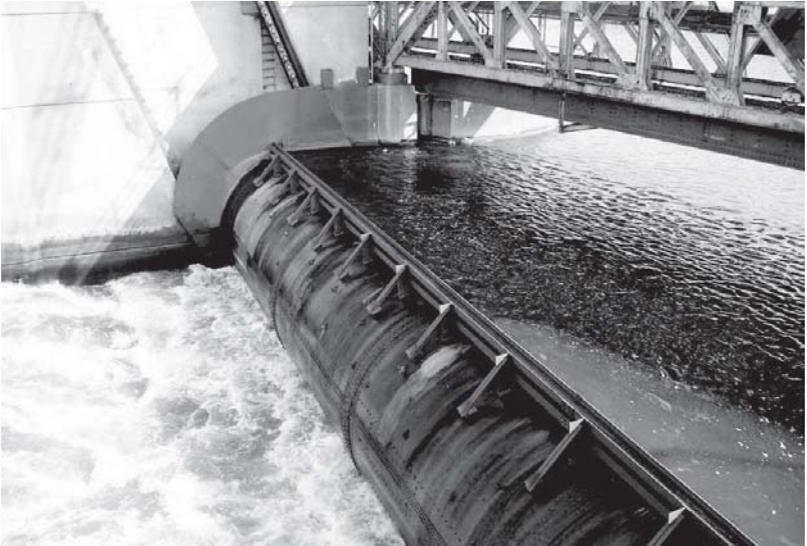
Figure 2-33. Roller dam gate (Courtesy of USACE).
