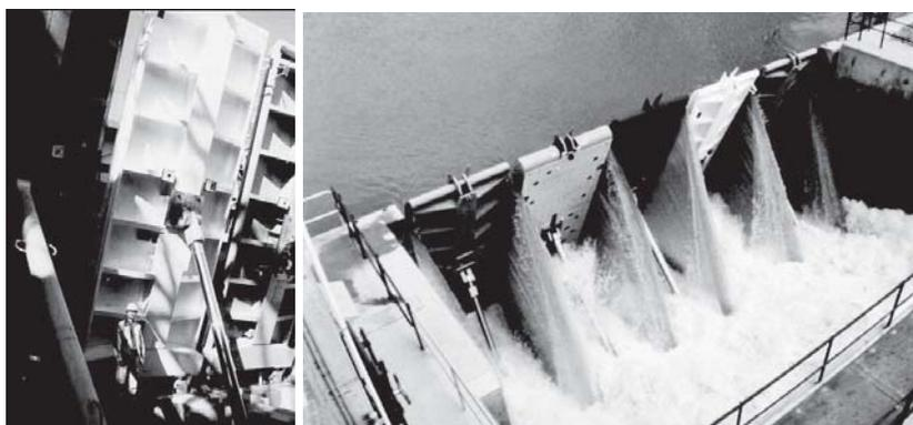
Figure 2-21. Hydraulically actuated wicket gates
