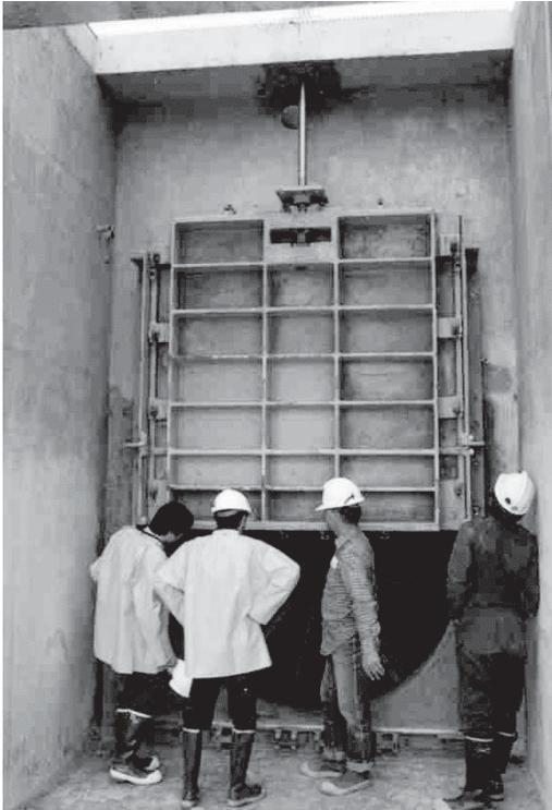
Figure 2-47. Sluice gate outlet work
