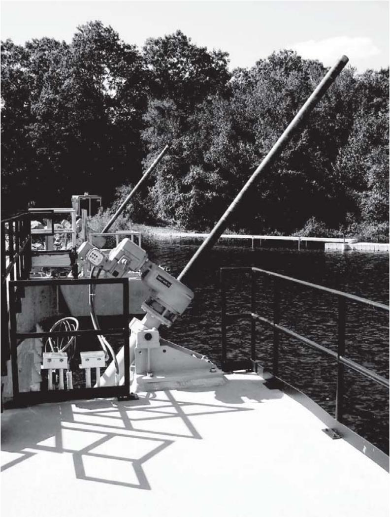
Figure 2-69. Screw stem gate operator.
