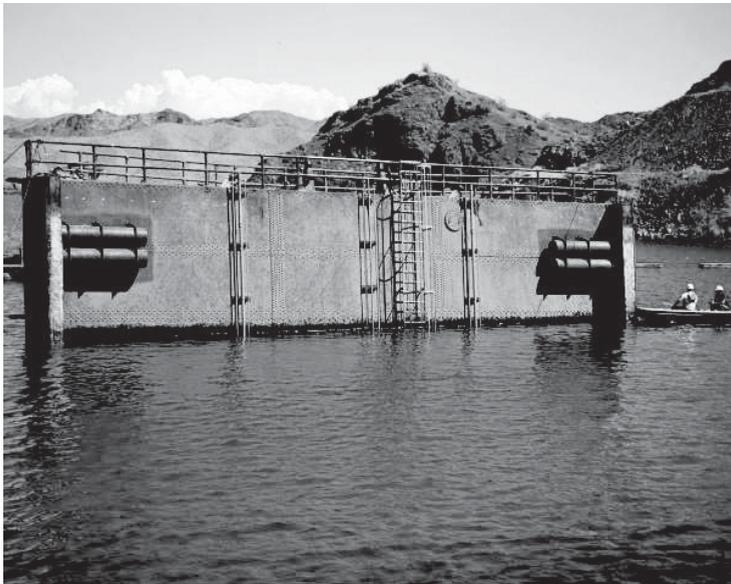
Figure 2-23. Single-piece floating bulkhead being positioned.
