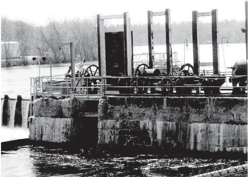
Figure 2-68. Rack and pinion gate operator.
