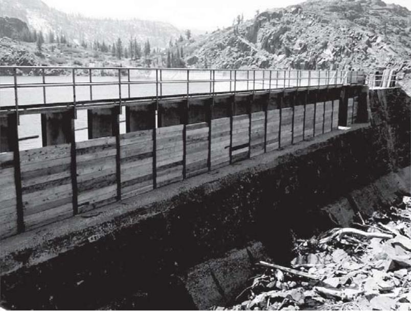
Figure 2-16. Fixed frame flashboards.
