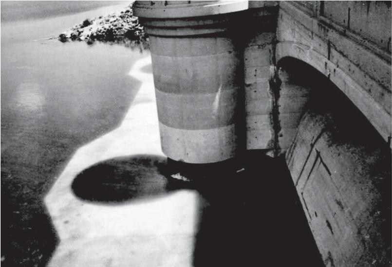
Figure 2-54. Intake with operating cylinder gate (Courtesy of USBR).
