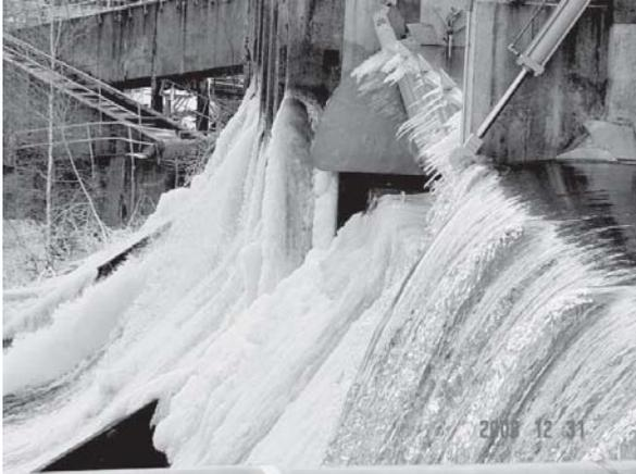
Figure 3-3. Icing of spillway gates.
