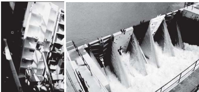
Figure 2-21. Hydraulically actuated wicket gates
