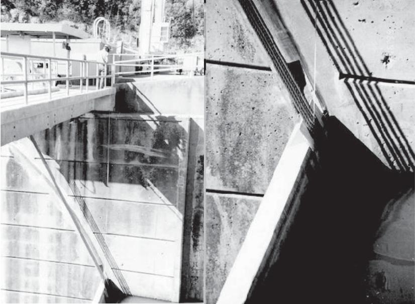
Figure 8-1. Tainter gate non-uniform lift misalignment measurement.
