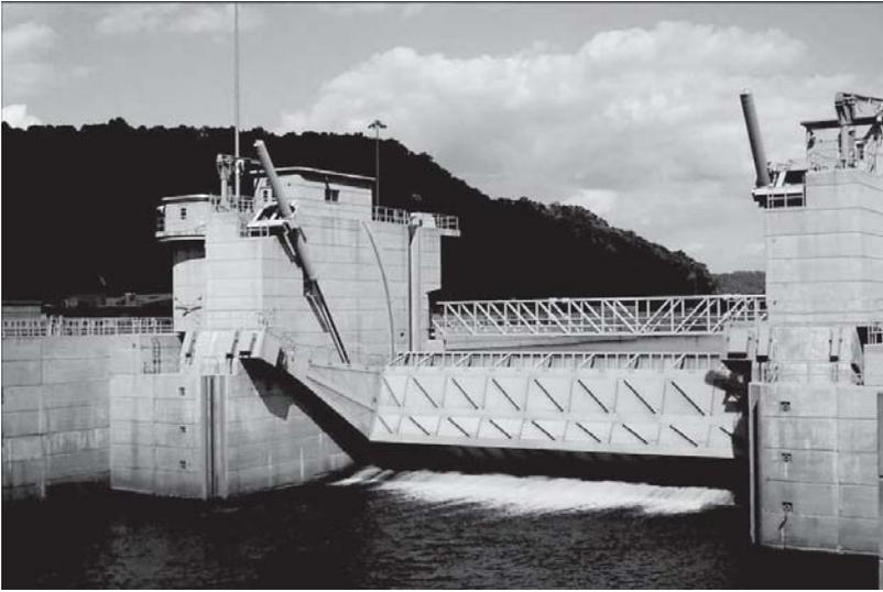
Figure 2-70. Radial gate with hydraulic cylinder actuator (Courtesy of USACE).
