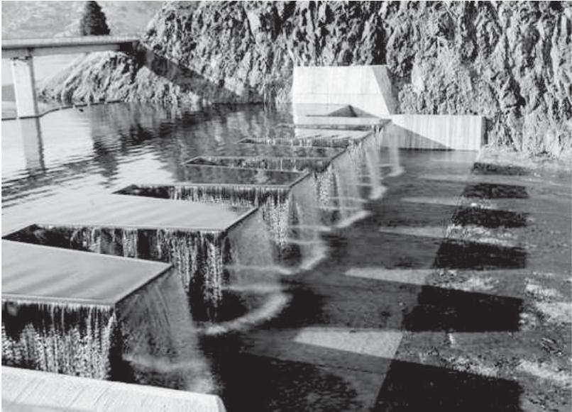
Figure 2-57. Labyrinth fuse gate (Courtesy of USBR).
