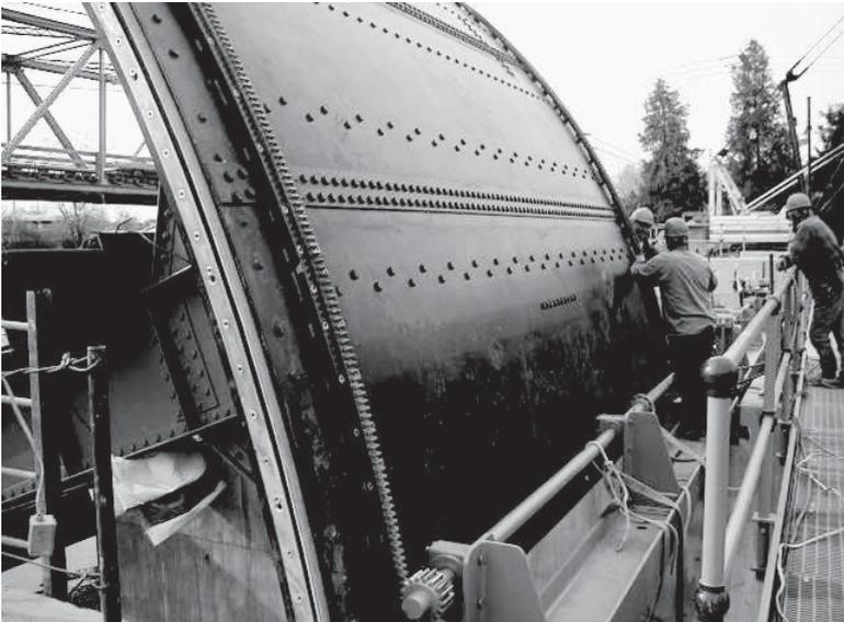
Figure 2-67. Rack and pinion gate operator.
