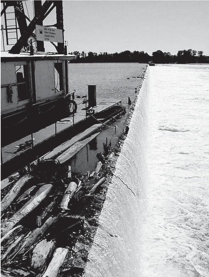
Figure 2-19. Wicket gates (manual placement type)
