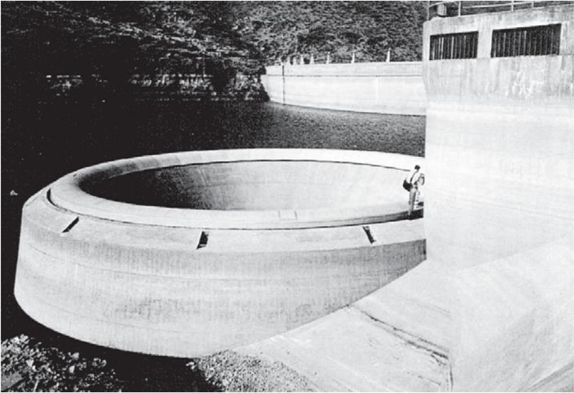
Figure 2-55. Ring gate (Courtesy of USBR).
