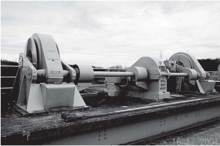
Figure 2-60. Drive, reduction gears, drums, and connection shafts (Courtesy of TVA).
