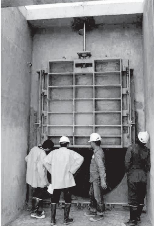
Figure 2-47. Sluice gate outlet work
