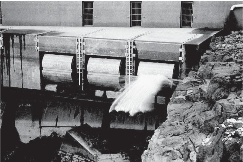
Figure 2-52. Clamshell gate after installation (Courtesy of USBR).
