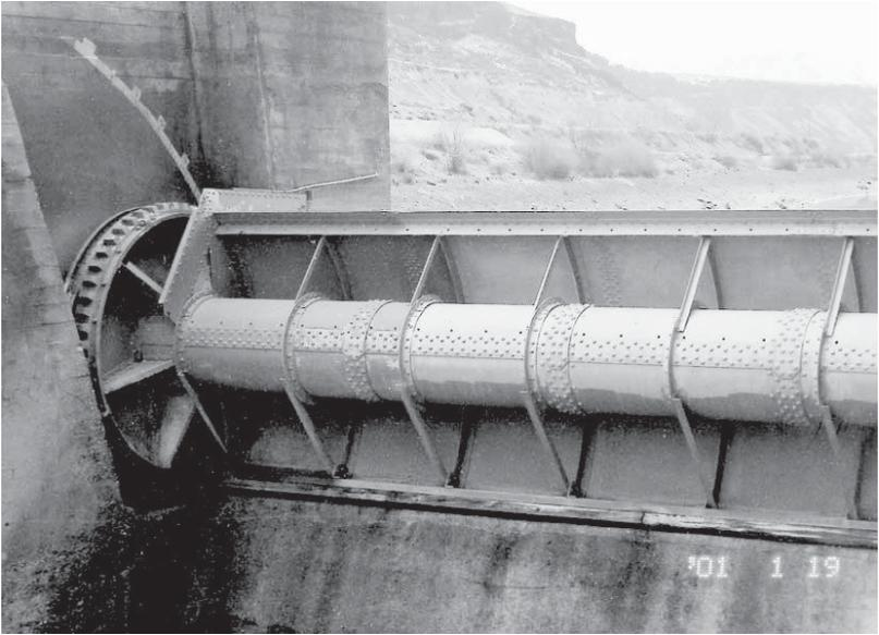
Figure 2-32. Non-submersible roller dam gate (Courtesy of USBR).
