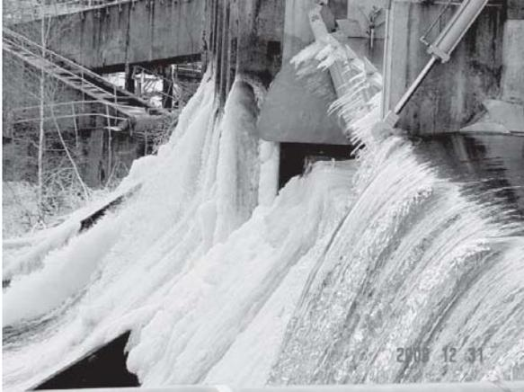
Figure 3-3. Icing of spillway gates.
