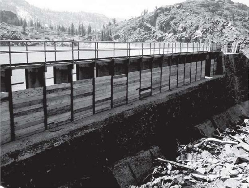
Figure 2-16. Fixed frame flashboards.
