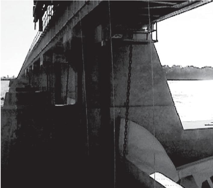
Figure 2-66. Link Chain (Courtesy of USACE).
