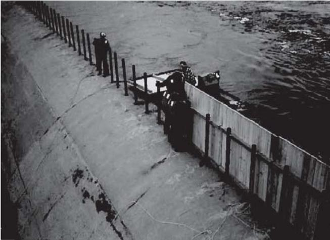
Figure 2-13. Installation of pinned flashboards.
