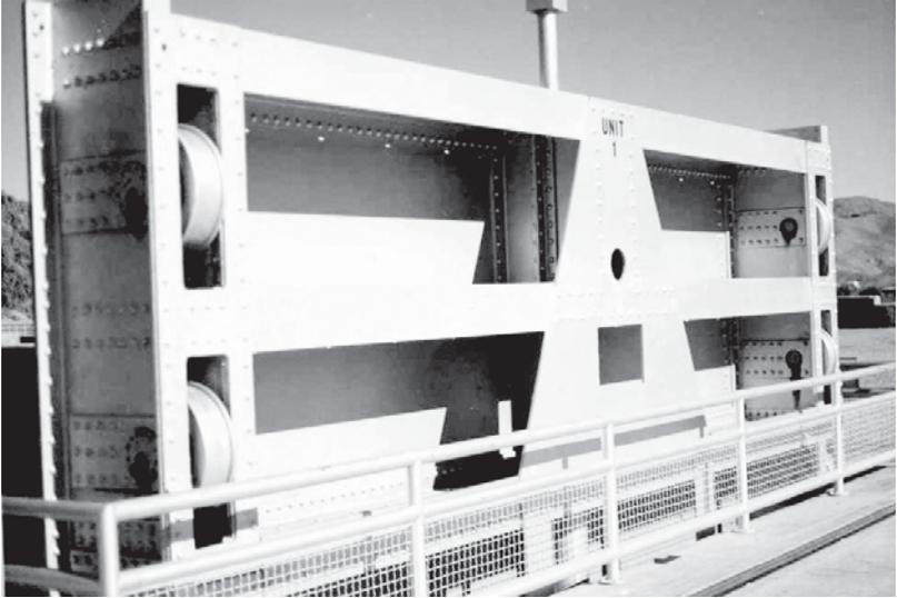
Figure 2-35. Wheel-mounted gate (Courtesy of USBR).
