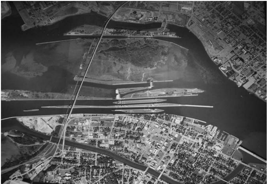
Figure 5.8 Lake Superior Control Works at Sault Ste. Marie, Ontario/Michigan.
