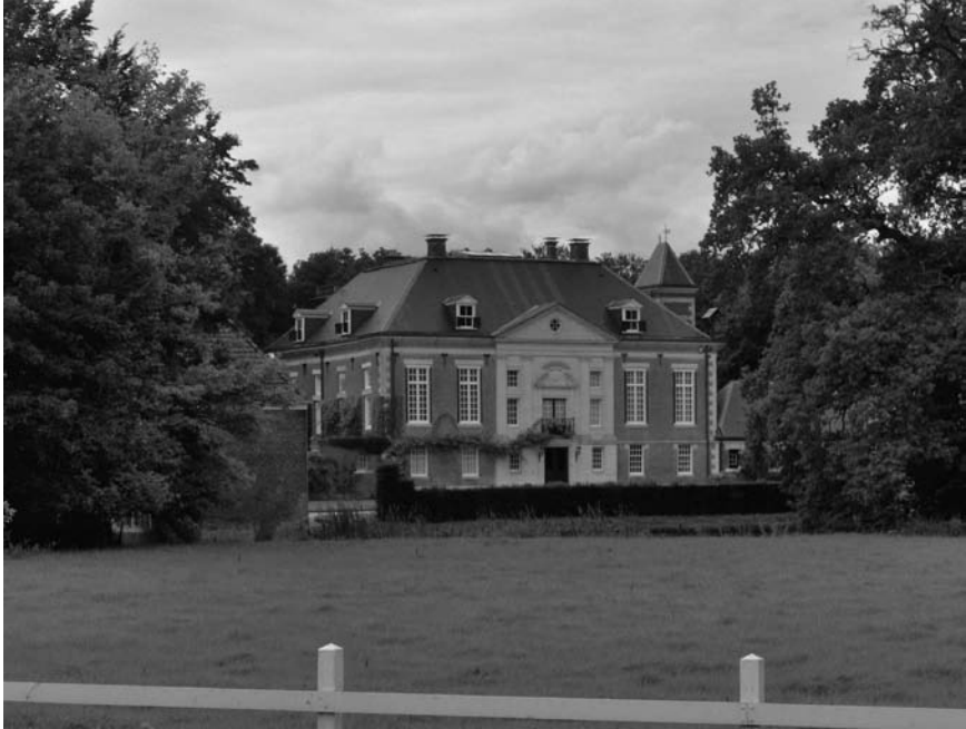
Figure 11.4 One of the estates: House of Diepenheim.
