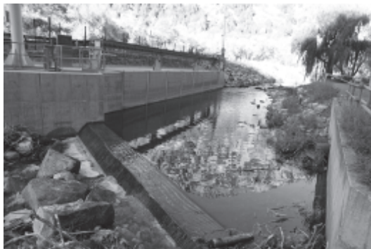
Fig. 7. Example of a flow diversion structure (photo courtesy of Blake Tullis).
