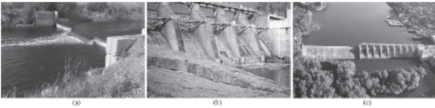
Fig. 6. Example of parallel flow control structures: (a) staged linear weir (photo courtesy of Steven Barfuss); (b) ogee crest weir with radial gates (Wirtz dam, TX, USA) (photo courtesy of Blake Tullis); (c) parallel gated and non-gated ogee crest spillways (Tom Miller Dam, TX, USA, photo courtesy of Freese and Nichols Inc.).
