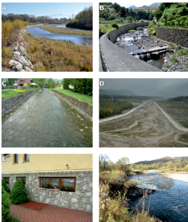
Fig. 3. Examples of mountain channel regulation structures and other anthropopressure: A – Longitudinal regulations (Czarny Dunajec River, Poland), B – Transversal regulations (Ribeira do Grande, Madera), C – Artificial trough (Krośnica Stream, Poland), D – Channel narrowed due to regulation (Liyuan-He, China), E – Large boulders used for building purposes (Podhale region, Poland), F – Channel with remaining elements of training structures (Skawa River, Poland).
