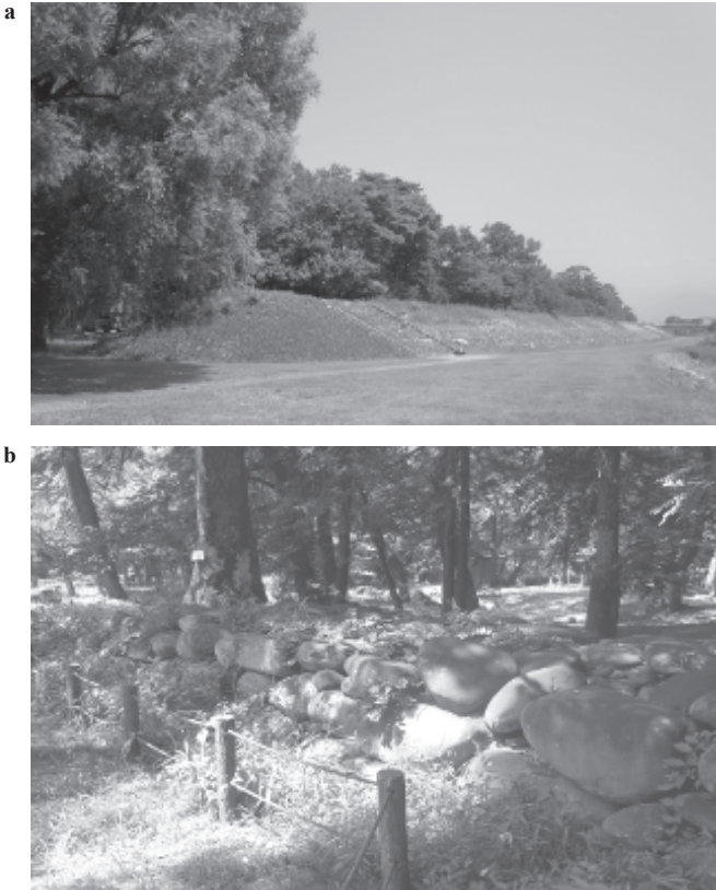
Photo 1. Flood protection forest “Manriki Forest (Mighty Forest)”. (a) A view from floodplain, (b) Rubble mound dyke in the forest
