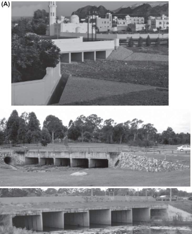
Fig. 8. Box culverts. (A) Muscat, Oman on 31 Oct. 2010 afternoon; (B) Culvert outlet below Ridgewood St, Algester (QLD, Australia) in August 1999; (C) Culvert along Gin House Creek, Carrara, Gold Coast (QLD, Australia) on 5 Dec. 2007.
