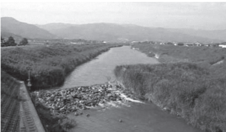
Photo 2. Rubble mound weir in Jobaru River. (Kyushu Regional Development Bureau, Ministry of Land, Infrastructure, Transport and Tourism, MLIT, Japan.)
