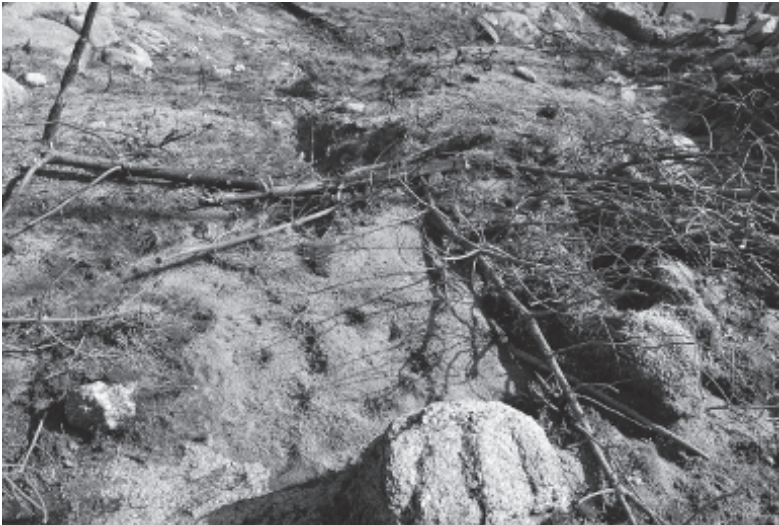
Photo 11. Accumulation of sediments in barriers made from the remains of burnt pines and pine needles.
