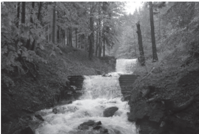
Fig. 5. Wooden and concrete check-dam structures during higher flow event with ca. 2 year recurrence interval (the Malá Ráztoka Stream, Western Carpathians, Czech Republic).
