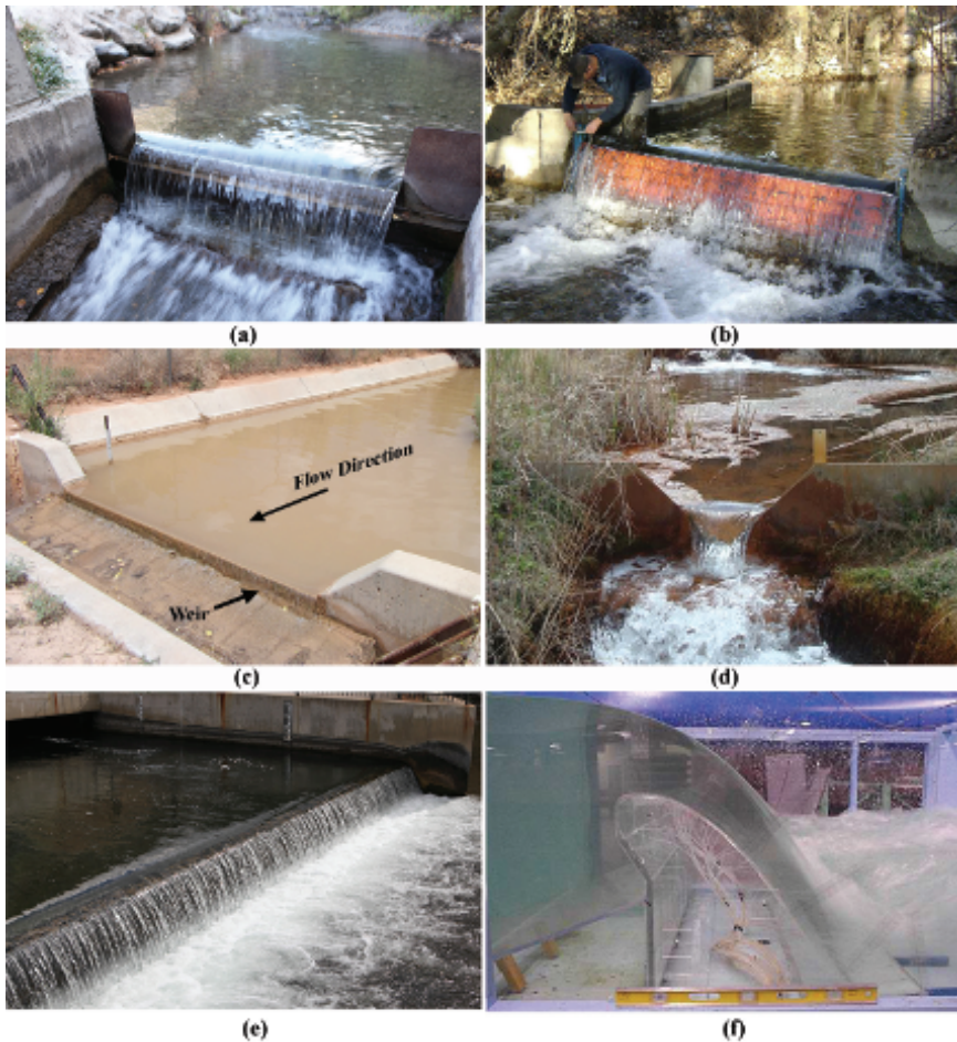
Fig. 1. Examples of various linear weir types: (a) contracted rectangular (sharp-crested) weir (photo courtesy of Blake Tullis), (b) rectangular (sharp-crested) weir (photo courtesy of Blake Tullis), (c) Cipoletti (flattop) weir (photo courtesy of Steven Barfuss), (d) V-notch (sharp-crested) weir (Photo courtesy of Bret Dixon), (e) suppressed rectangular (flattop) weir (photo courtesy of Blake Tullis), (f) ogee crest weir (photo courtesy of Blake Tullis).
