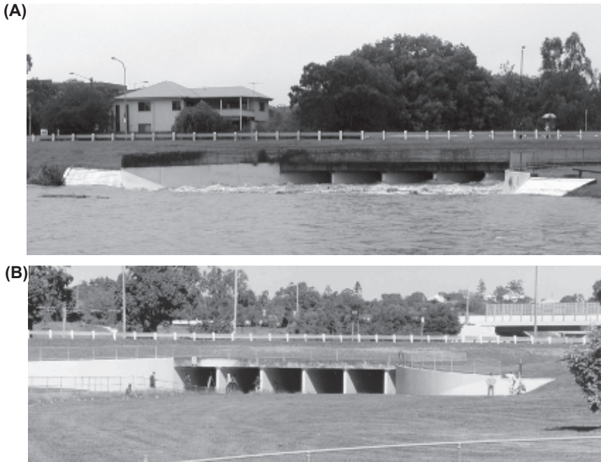
Fig. 9. Minimum energy loss culvert along Norman Creek beneath Ridge Street, Brisbane (Australia). (A) Inlet operation on 7 Nov. 2004 for Q \approx 80 to 100 \text{ m}^3/\text{s} ; (B) Outlet on 13 May 2002.
