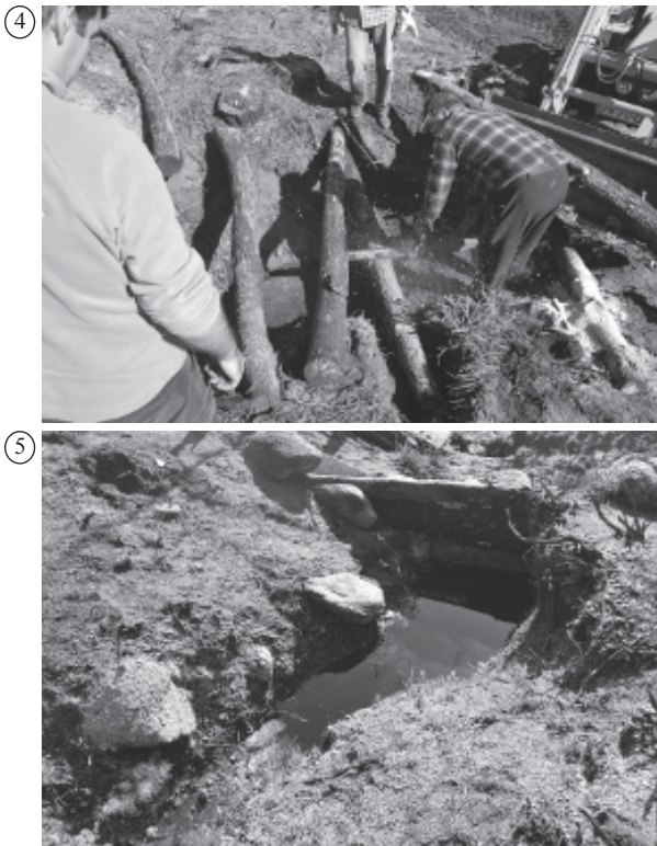
Photos 4 and 5. Construction of log check dams.
