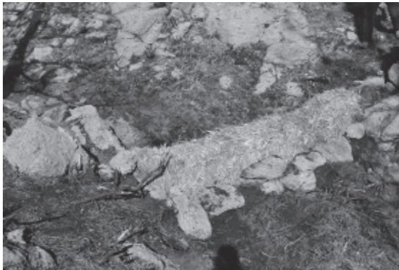
Photos 6 and 7. Straw bale barrier implemented.
