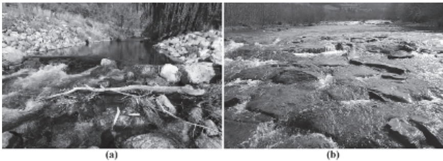
Fig. 9. Block or rock ramp grade control structures in river applications: (a) single rock ramp structure (photo courtesy of Blake Tullis); (b) two rock ramps in series (photo courtesy of Artur Radecki-Pawlik).
