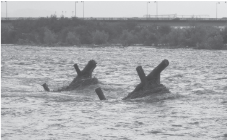
Photo 3. Crib spur fighting against flood flow in 2011. (Photo taken by Kofu River and National Highway Office, Kanto Regional Development Bureau, MLIT.)
