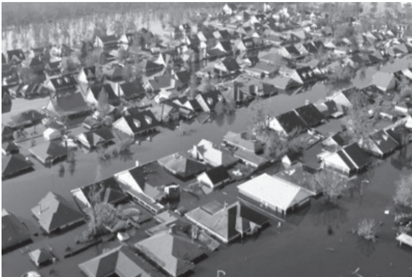
Fig. 2. Flooding in New Orleans, USA (August 2005) by failure of defense against floods.
