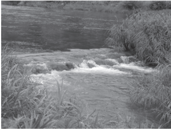
Photo 5. Rough ramp in Maruyama River, Japan.
