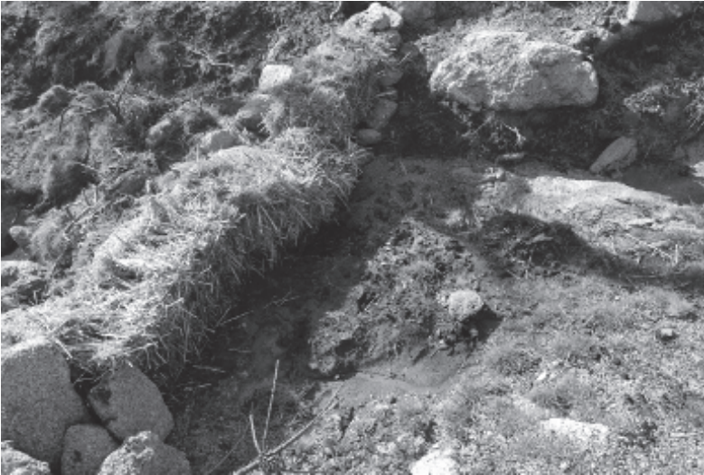
Photo 10. Accumulation of sediments in a straw bale barrier.
