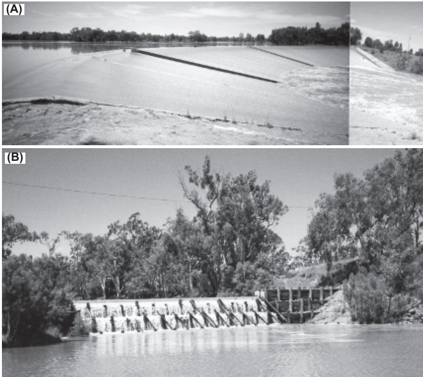
Fig. 2. Unusual weir designs in Australia: (A) Minimum energy loss weir on the Condamine River (Chinchilla, QLD); (B) Timber crib weir on MacIntyre Brook (Whetstone weir, QLD).
