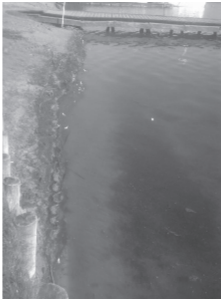
Fig. 11. The process of cyanobacteria bloom formation as a result of great concentrations of phosphates in the groundwater and their input to the human-transformed littoral zone (photo by M. Zalewski).
