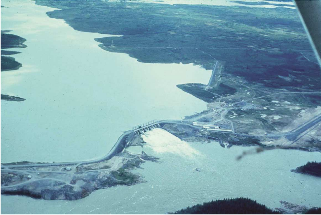
FIGURE 19.9 The Kettle Rapids dam on the Lower Nelson River was the first of a series of dams that have flooded out the rapids and divided the deeply incised river channel into a series of flooded valley reservoirs. Ice damming and ice jams no longer occur (PHOTO BY R. NEWBURY).
