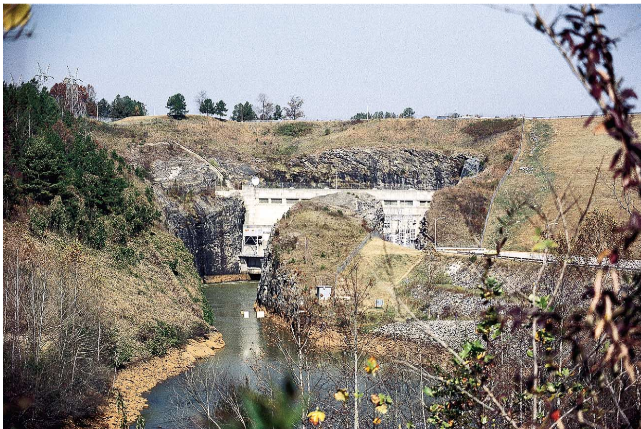
FIGURE 4.4 Chattahoochee River (Apalachicola system) below Buford Dam (Lake Lanier), north of Atlanta. Note tan waterline on cliffs indicates daily/weekly fluctuations in water level from hydropower releases (PHOTO BY A. C. BENKE).
