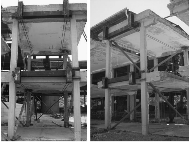
Figure 4.35 The RC structure equipped with BRBs.
