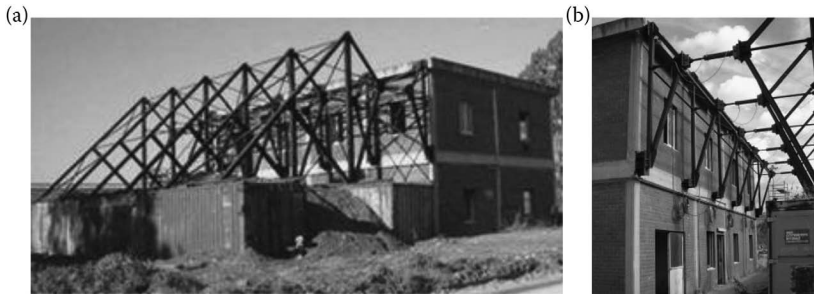
Figure 4.42 Reacting structure (a) and hydraulic jacks (b).
