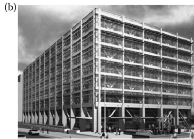
Figure 4.30 Wallace F. Bennett Federal Building (USA): before (a) and after (b) seismic retrofitting.
