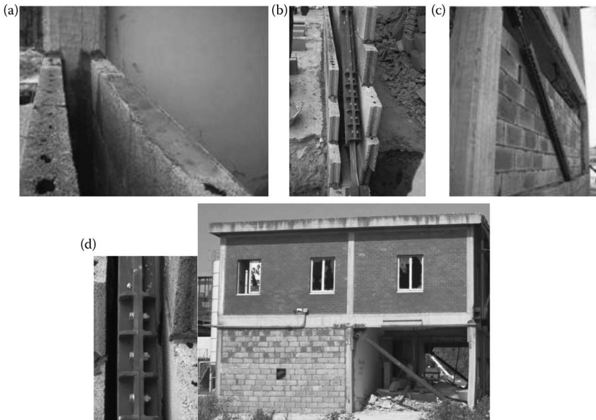
Figure 4.41 Intermediate erection phases (a,b,c) and the final configuration (d).
