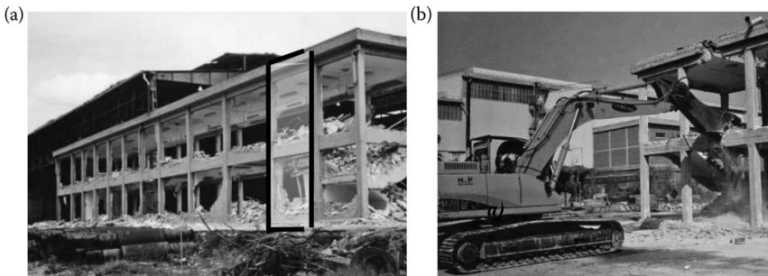
Figure 4.99 The original RC building after the partition removal (a) and subdivision in separate modules (b).
