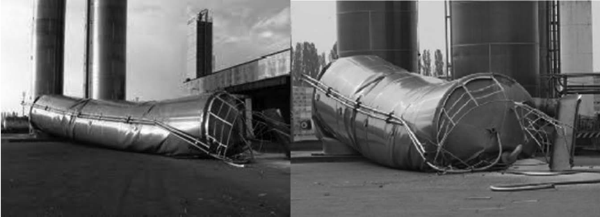
Figure 1.67 The collapse of a steel silo during the Emilia earthquake. (Faggiano, B. et al. 2012: Steel buildings within the Emilia earthquake (in Italian). Progettazione Sismica , n.3, IUSS Press, ISSN 1973–7432.)
