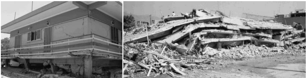
Figure 2.11 Typical collapses of frame buildings with open ground storey; ‘pancake’ type of collapse shown on the right.
