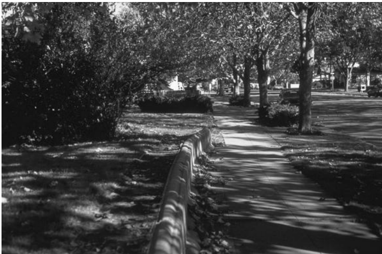
Figure 2.4 Fence offset in Hollister, California.
