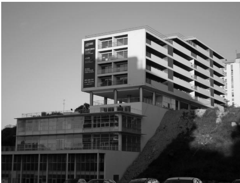
Figure 4.5 Example of an irregular building.
