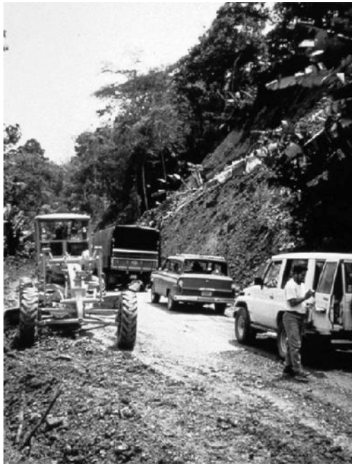
Figure 2.29 Slope failure on State Highway 17, California (Loma Prieta earthquake, 1989).
