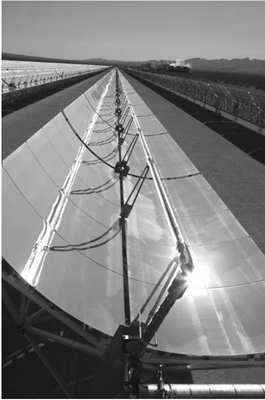
Fig. 13.6 A solar thermoelectric system. Solar concentrator mirrors and tube system. (Photograph of ACCIONA's Nevada Solar One courtesy of ACCIONA)
