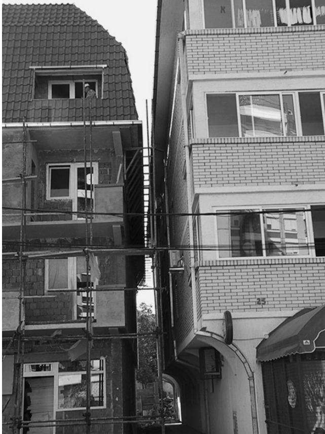
Fig. 18.1 Illegal construction in Belgrade
