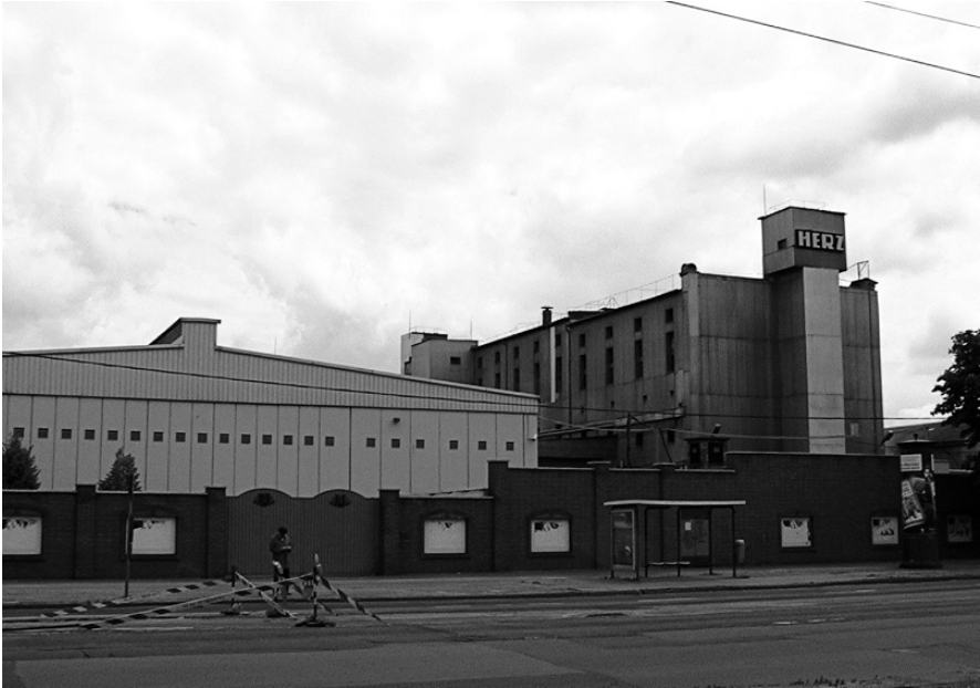
Fig. 8.5 The Herz meat factory. One of the largest food processing factories in Hungary is situated in the southern industrial district of the city. Within the old factory gates, significant redevelopment took place in the 1990s
