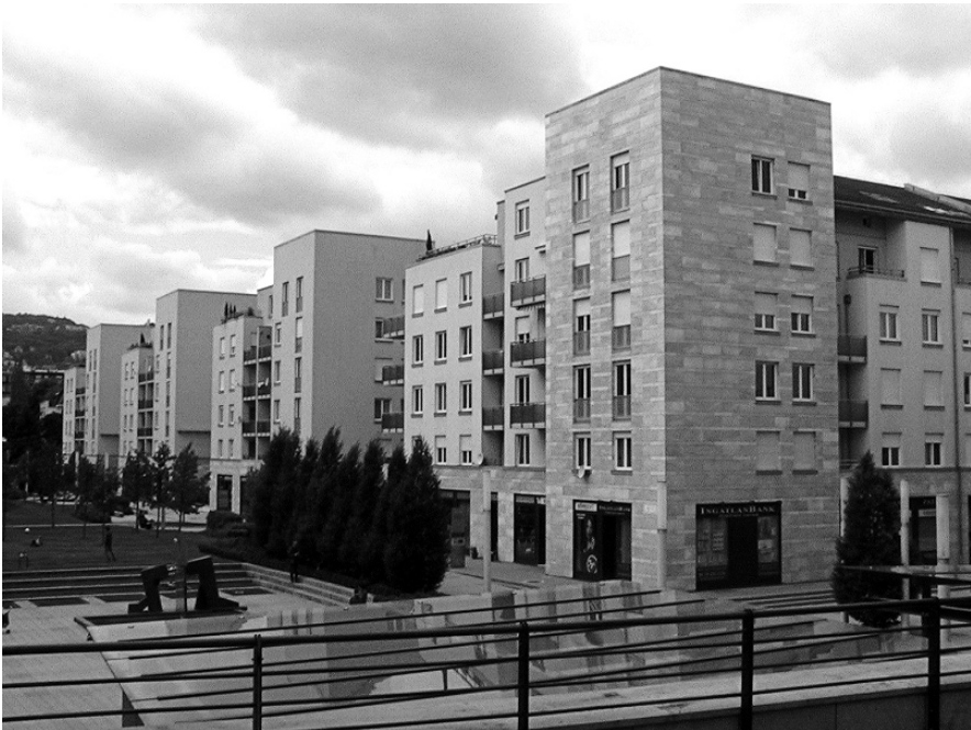
Fig. 8.11 The MOM residential park. This prestigious development was built on the site of a former optical factory in 2002
