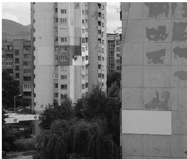
Fig. 11.6 Building renovations in the housing estate Mladost 3, Sofia
