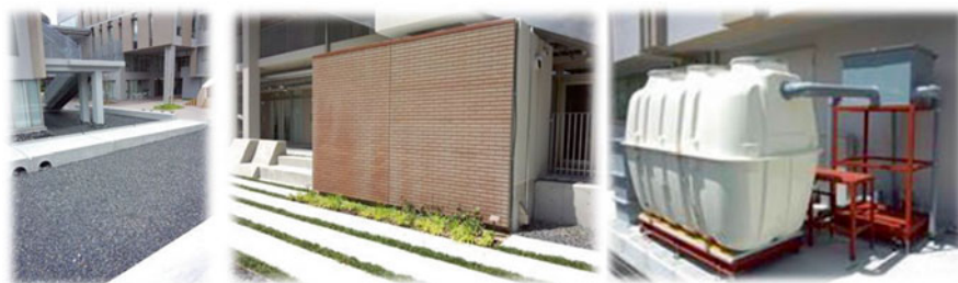
Fig. 11.4 Left: Environmental pond for rainwater storage (no water on fine days). Center: Plant irrigation wall. Right: Jokaso (treatment facility for greywater from the building)
