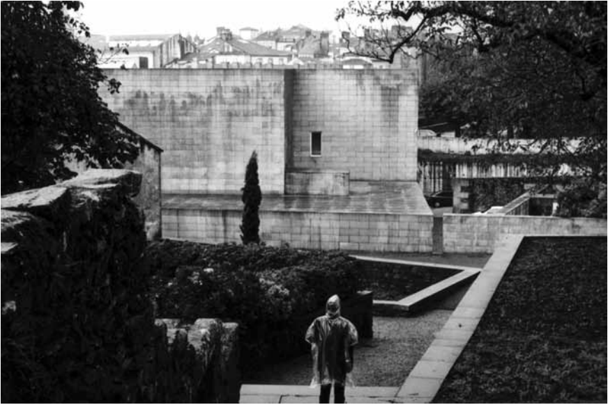
Figure 8.6 The Galician Centre for Contemporary Art, looking west from the convent garden with distant views of the spires and domes of the Cathedral of Santiago above the roof-line (photo by Claudia Lynch)
