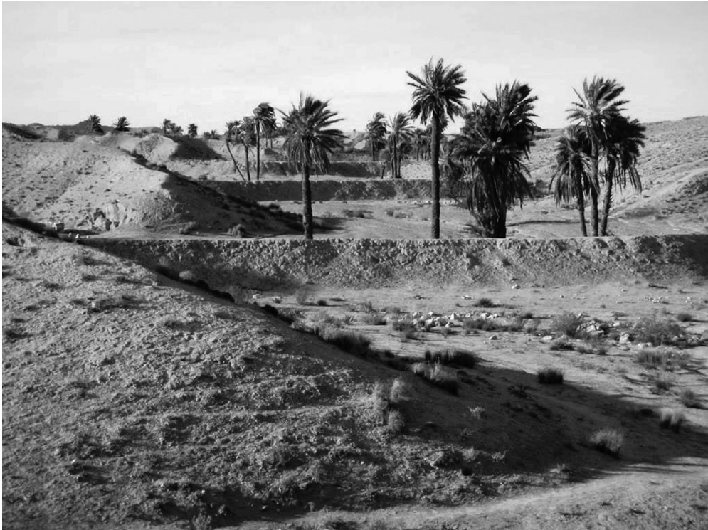
Figure 6.15 Soil and water conservation structures built across an ephemeral channel in loess at Matmata, Tunisia. (ASG)
