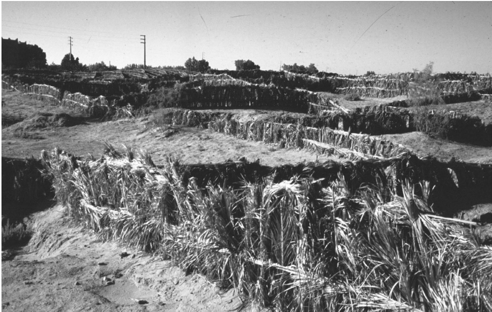
Figure 6.5 Checkerboard palm frond dune-control structures at Erfoud, Morocco. (ASG)
