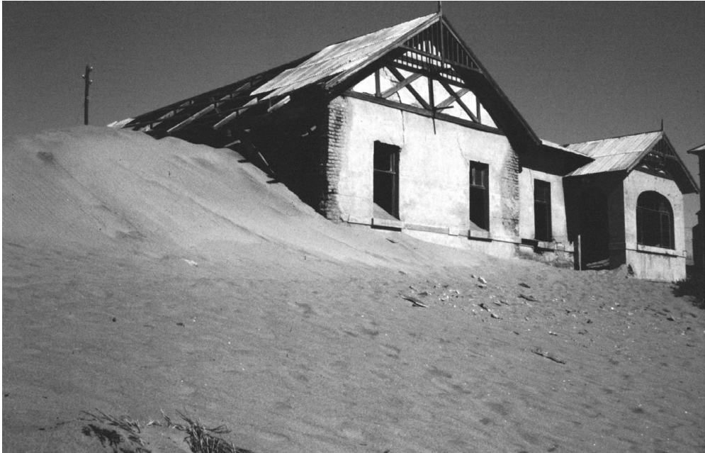
Figure 6.3 Sand encroaching on mining buildings at Kolmanskop, southern Namibia. (ASG)
