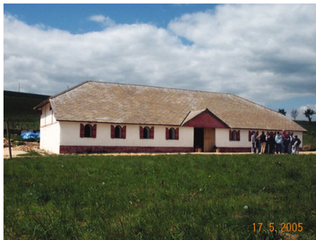
Experimental Geoarchaeology, Figure 4 Butser Experimental Romano-British Farm, Hampshire, UK; reconstructed Roman villa (designed from Sparsholt, near Winchester); a two-storied structure with load-bearing lime mortared flint walls and an upper story which is timber-framed with wattle and daub panels. Walls were lime plastered, floors were either mortared or made up of opus signinum to be more hard wearing; here crushed brick or terra-cotta was added to the mortar (see Figures 5, 6, and 7). ( http://www.butser.org.uk/bulletin30.html ; Christine Shaw, pers. comm).
