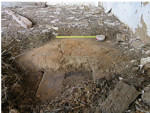
Ethnogeography, Figure 1 Photograph showing a section dug into the clay floor of an abandoned house at Sarakini, Greece. Thick oak beams forming the base are covered by a mud mixture and then overlain by successive clay laminae that represent floor replasterings. The loose sediment on the floor reflects debris accumulated after abandonment as well as secondary use remains (rye straw).
