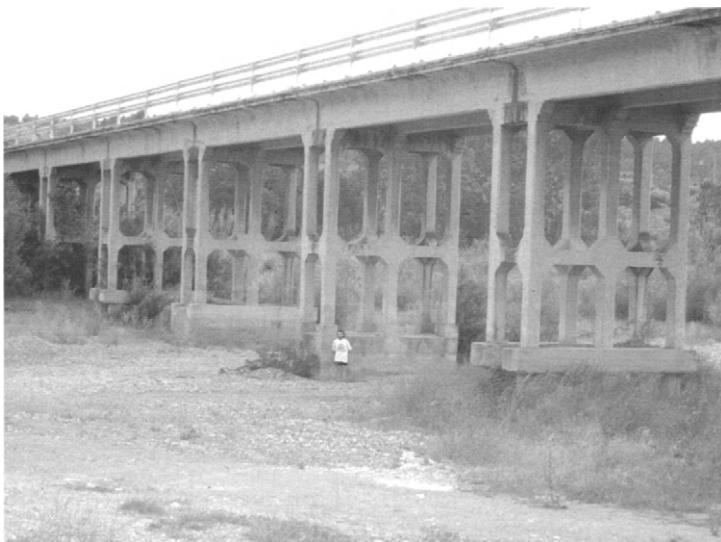
Figure 8. Bridge undermining due to gravel extraction in the Siurana River, Spain, upstream of the confluence with the Ebro River, NE Spain (photo: R.J. Batalla, June 2005)
