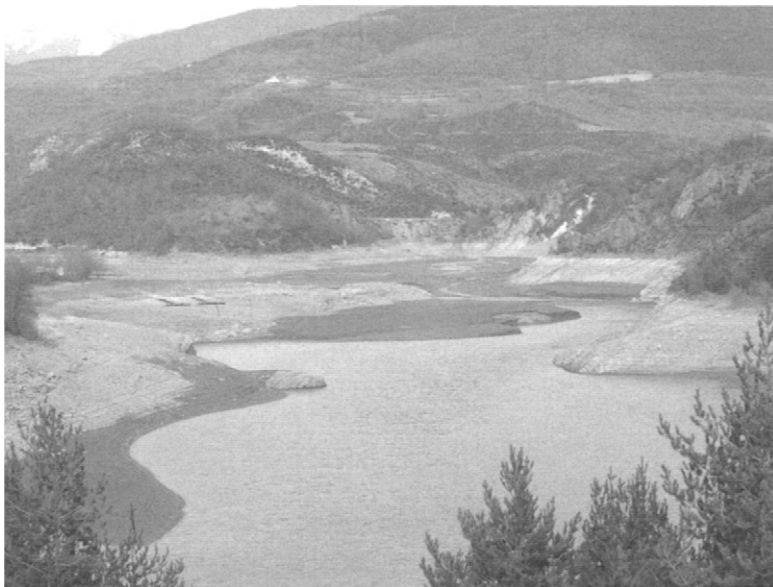
Figure 6. Sedimentation in the Escales Reservoir, Ebro River basin, Spain (photo: R.J. Batalla, February 2004)
