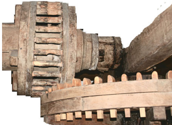
Fig. 6 Design and appearance of wooden gears after many years of in operation
