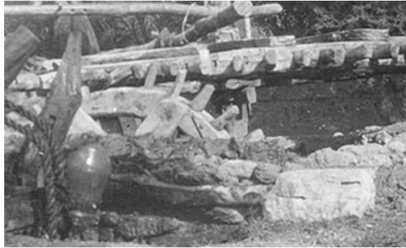
Fig. 2 Gearing of a sakia
