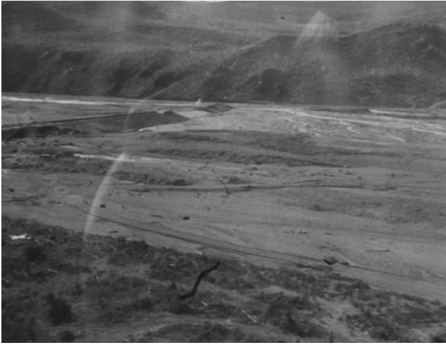
Figure 11-4. Breach of the N1 structure, Hoffstadt Creek near Mount St. Helens. Source: © MBH Software, Inc. Used with permission.
