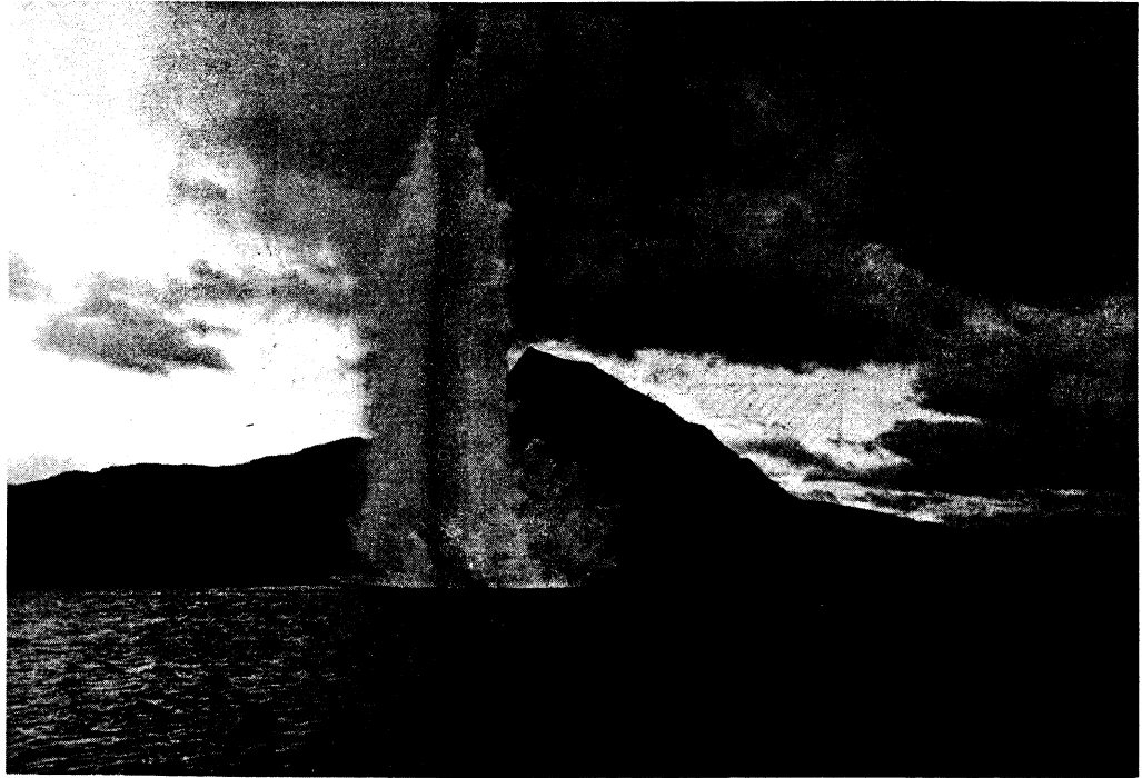
Water column after plug blasting.
