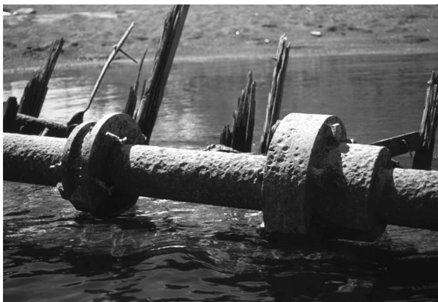
Fig. 2.60 View southeast of after bulkhead stuffing box and gland ( left ), and propeller shaft coupling ( right ). NPS photo by Brett Seymour
