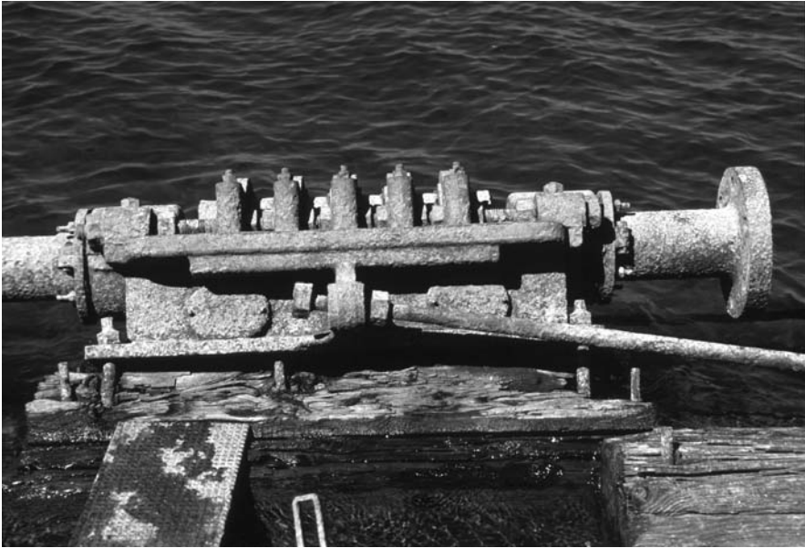
Fig. 2.57 Starboard side of thrust bearing. NPS photo by Jim Bradford
