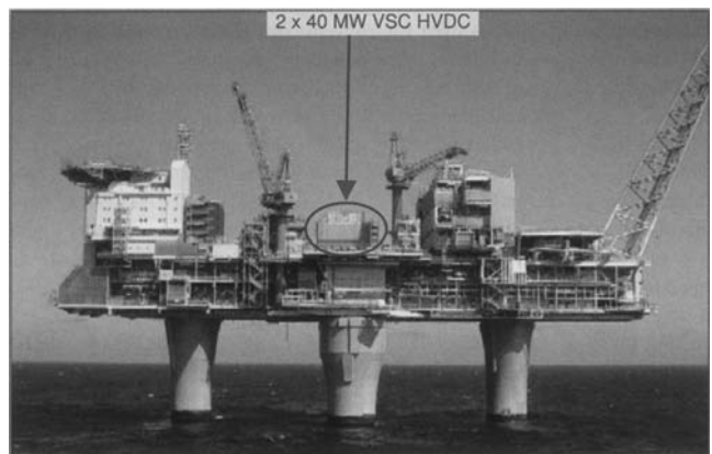
Figure 11 VSC power supply to Troll A production platform
