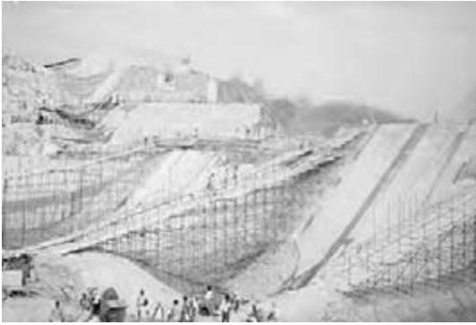
A major Indian dam and irrigation project under construction.
